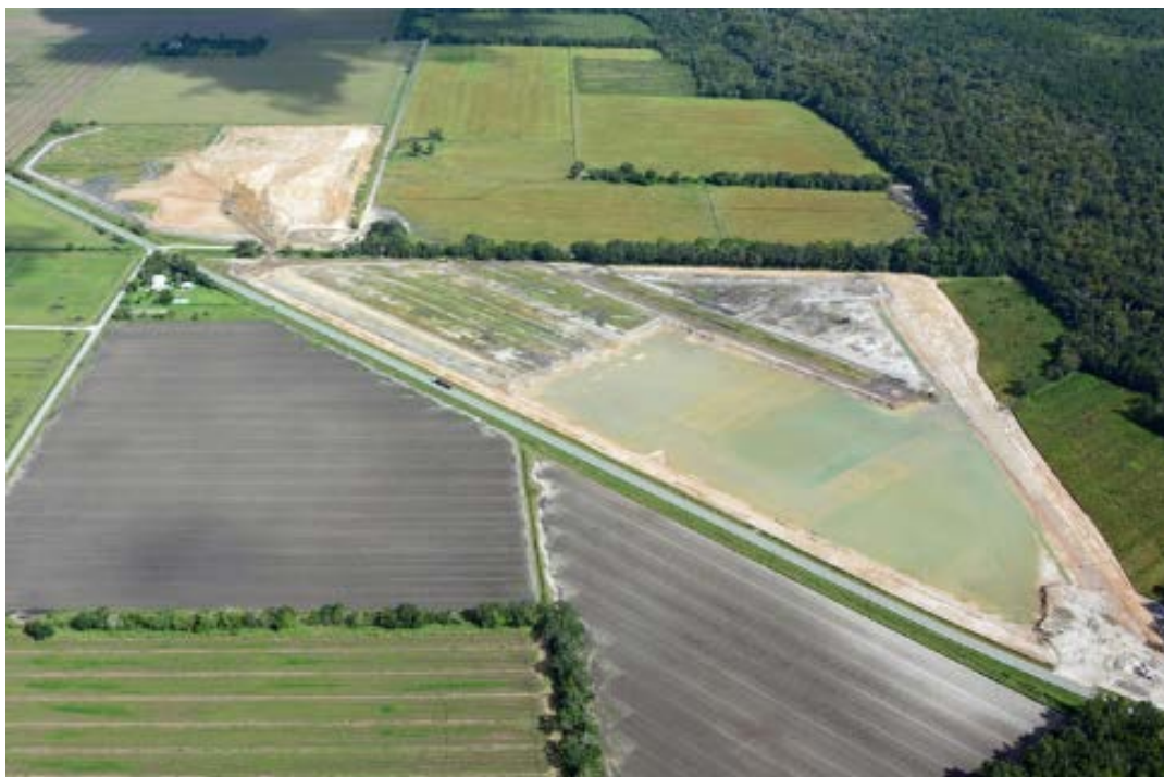
FIGURE 11: ST. JOHNS COUNTY MASTERS TRACT CONSTRUCTION IN SEPTEMBER 2013
