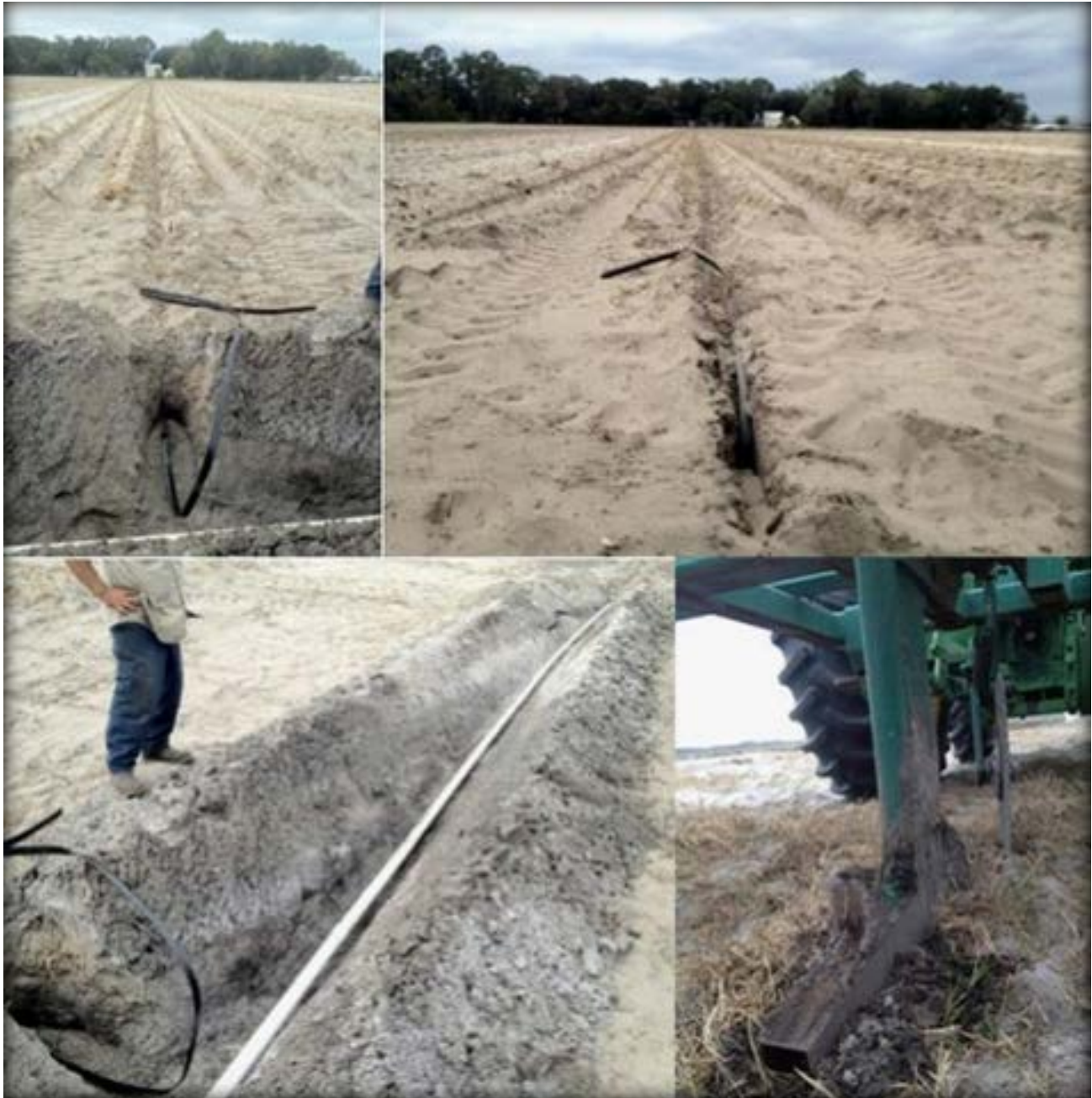
FIGURE 21: INSTALLATION OF SUBSURFACE DRIP TAPE
