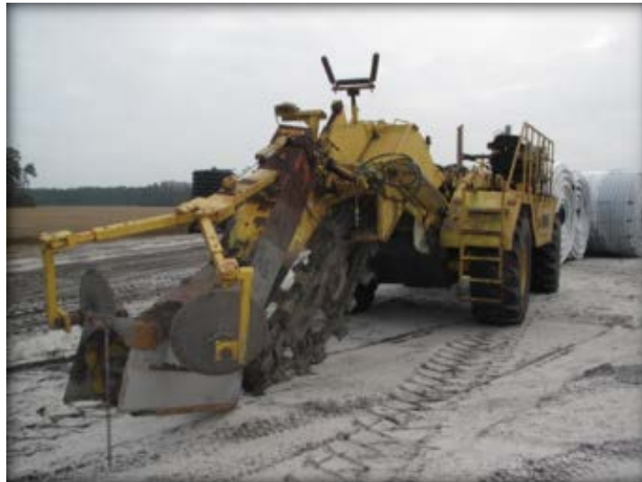
FIGURE 19: INSTALLATION OF IRRIDRAIN SYSTEM
