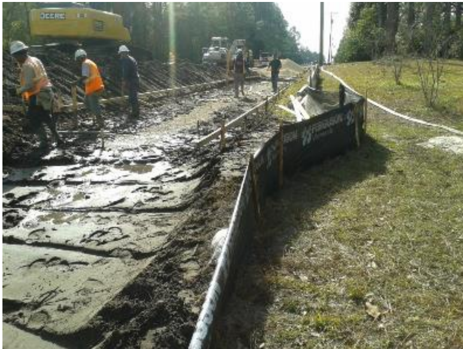
FIGURE 10: CLAY COUNTY CONSTRUCTION OF THE CR 739 WIDENING PROJECT
