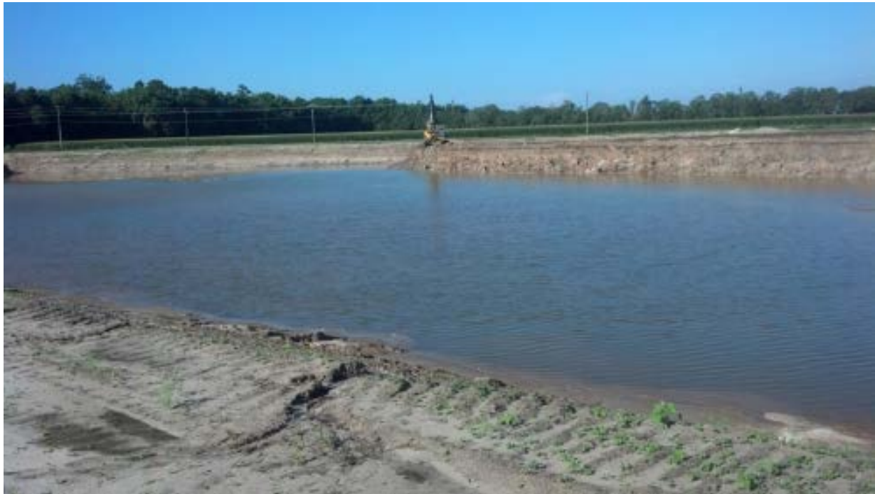
FIGURE 15: ST. JOHNS COUNTY WET DETENTION POND CONSTRUCTION AT MASTERS TRACT
