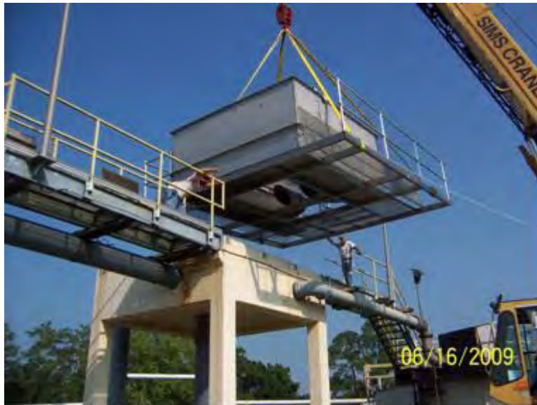
HOISTING MECHANICAL BARSCREEN CHANNEL INTO PLACE ATOP THE EXISTING SPLITTER BOX
