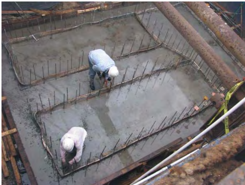
NEW BAR SCREEN FOUNDATION SLAB AFTER CONCRETE POUR WAS COMPLETED
