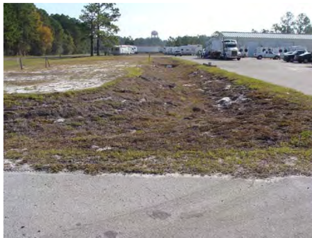
J6 OFFICE SWALE REPAIR
