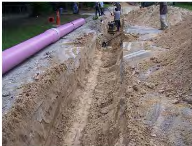
INSTALLATION OF 16-INCH PVC RECLAIMED WATER MAIN
