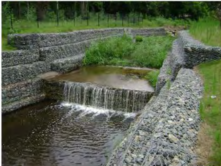
CITY OF JACKSONVILLE REGIONAL STORMWATER FACILITY OUTFALL
