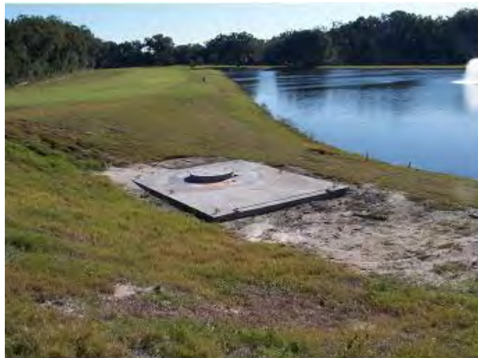
NEW RECLAIMED WATER PUMPING STATION BUILDING FOUNDATION
