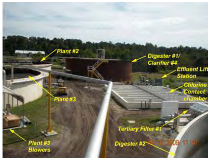
FIGURE 11: VIEW LOOKING EAST AT THE TOWN OF ORANGE PARK'S PROJECT AREA FROM DIGESTER #2
