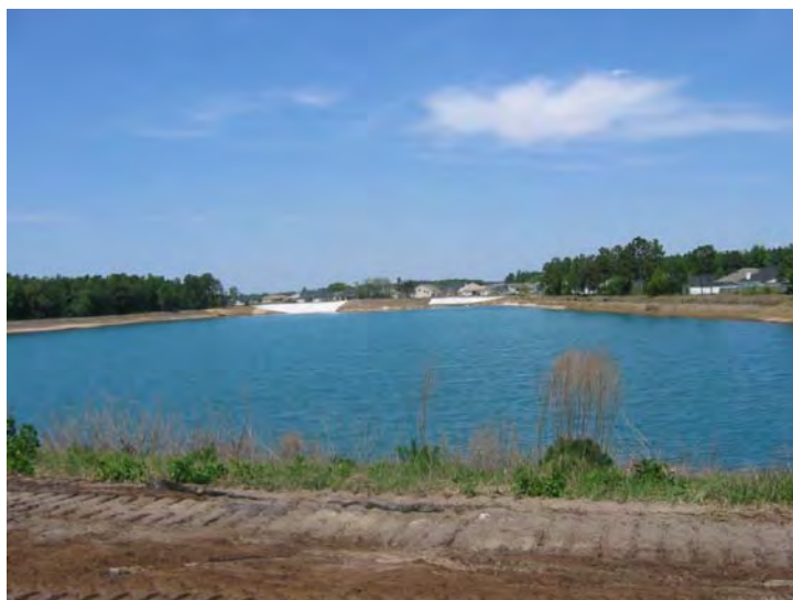
SANDALWOOD CANAL BORROW PIT STORMWATER FACILITY
