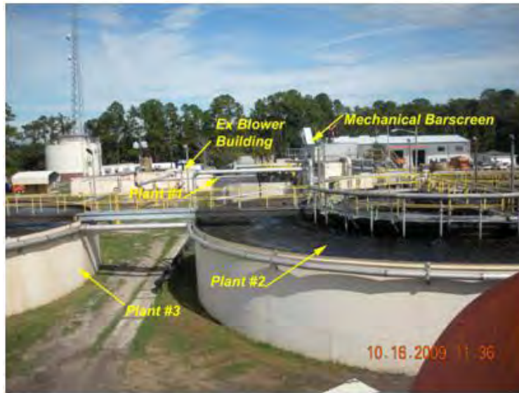
VIEW LOOKING NORTH AT PROJECT AREA FROM DIGESTER #1
