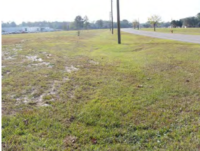
AVENUE A SWALE FROM JACKSONVILLE STREET
