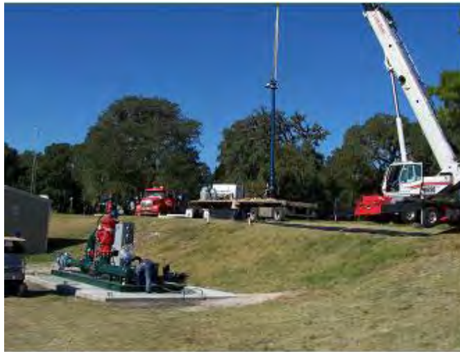
VERTICAL TURBINE PUMPS INSTALLATION
