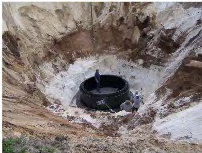
NEW PRE-CAST WET WELL INSTALLATION
