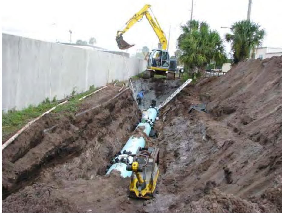
FIGURE 7: CITY OF JACKSONVILLE BEACH INSTALLATION OF NEW 24" EFFLUENT DISCHARGE PIPING FROM THE NEW CHLORINE CONTACT TANKS TO THE EXISTING EFFLUENT PUMP STATION
