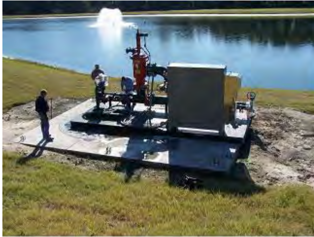
NEW RECLAIMED WATER PACKAGE PUMP SKID INSTALLATION
