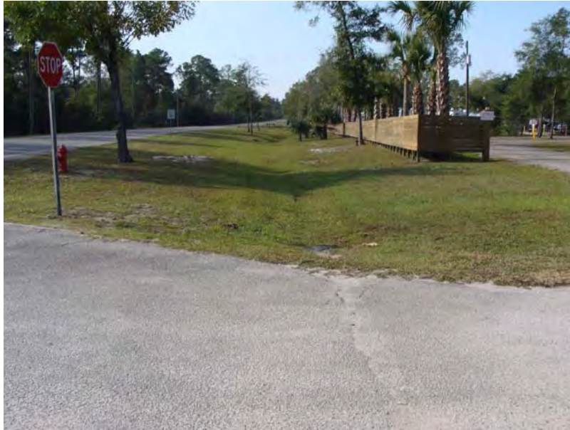
RV PARK SURFACE AREA DRAINAGE LOCATED ON AVENUE A SWALE
