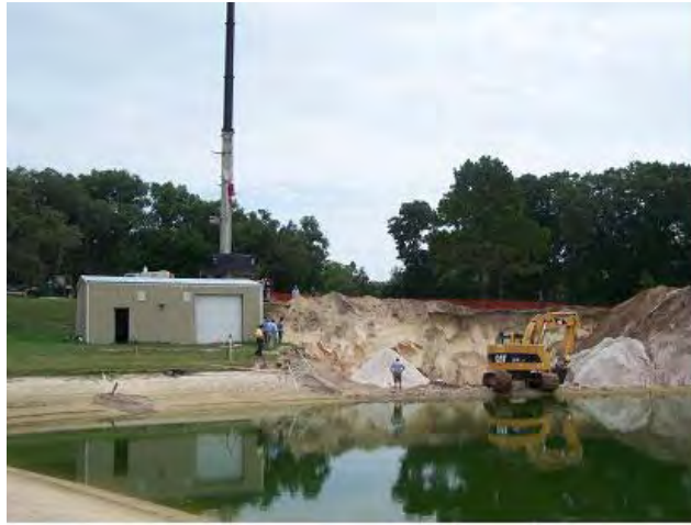
PRE-CAST WET WELL INSTALLATION AT GOLF COURSE RECLAIMED WATER HOLDING POND
