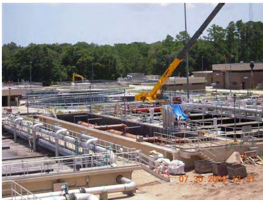
FIGURE 10: JEA ARLINGTON EAST WWTF CONSTRUCTION PROJECT
