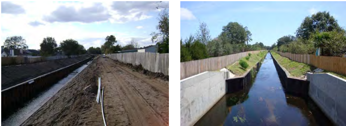
FIGURE 16: CITY OF JACKSONVILLE SANDALWOOD CANAL UNDER CONSTRUCTION (PHOTO AT LEFT) AND COMPLETED (PHOTO AT RIGHT)
