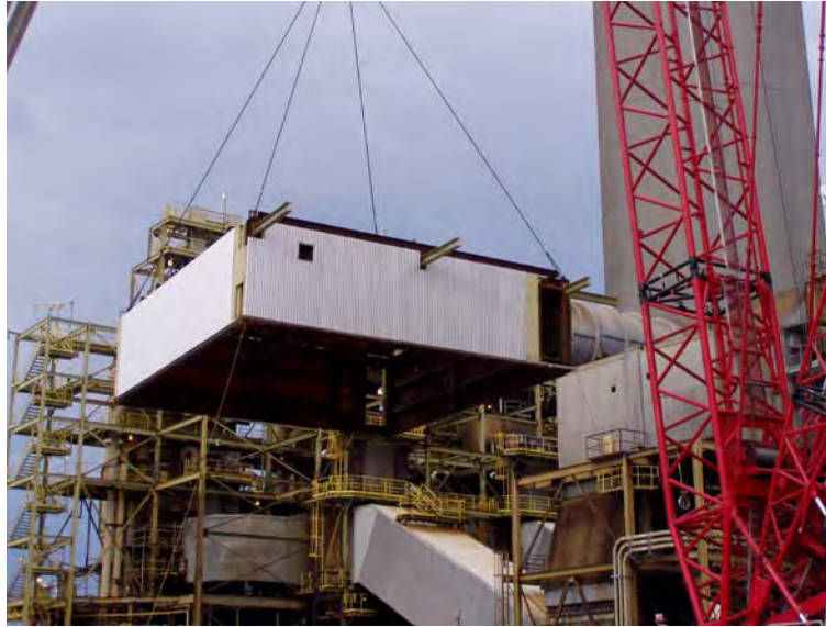
FIGURE 4: INSTALLATION OF SCR BOX
