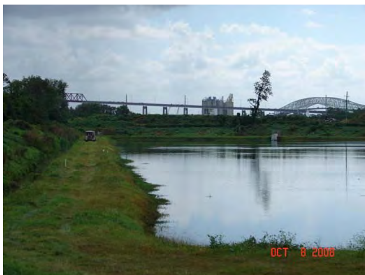
UPPER DEER CREEK REGIONAL STORMWATER FACILITY
