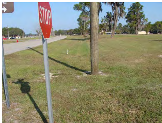
AVENUE A SWALE FROM JACKSONVILLE STREET
