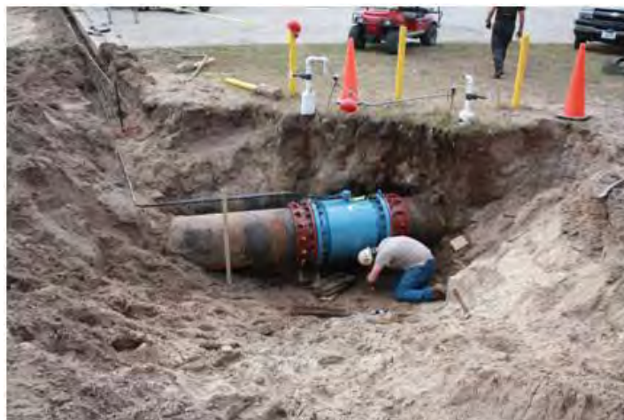
FIGURE 4: SEMINOLE ELECTRIC UPGRADES
