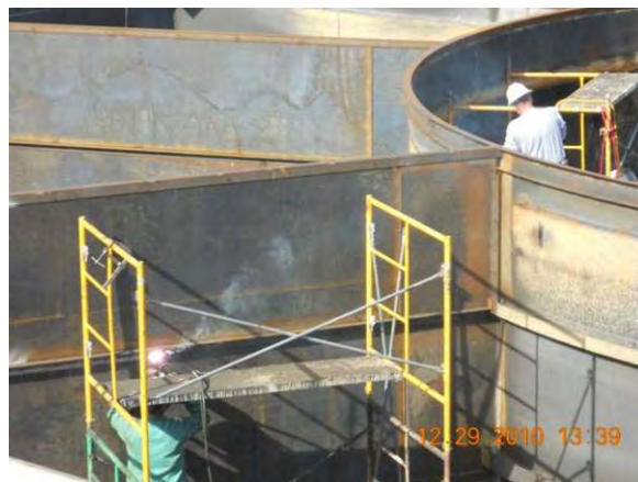
PBM CONSTRUCTORS, INC ERECT NEW STEEL BAFFLE WALLS
