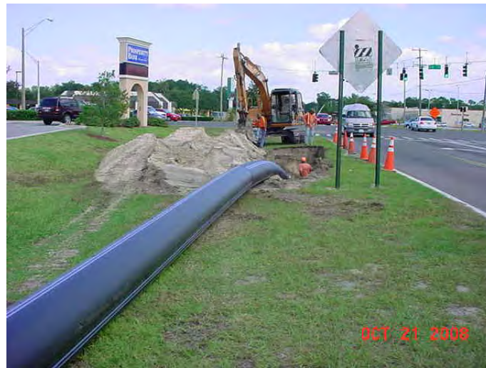
DIRECTIONAL BORE ON HIGHWAY 19
