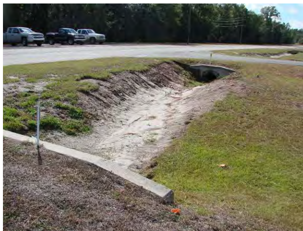
AVENUE D SWALE RECONSTRUCTION WITH NEW CULVERT PIPING (NOVEMBER 2010)
