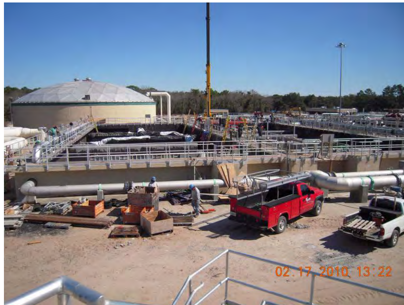
UPGRADES AT THE ARLINGTON EAST WWTF
