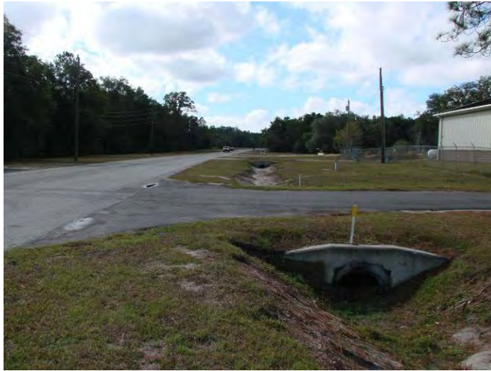
AVENUE D SWALE EXCAVATION AND REPAIR (NOVEMBER 2010)
