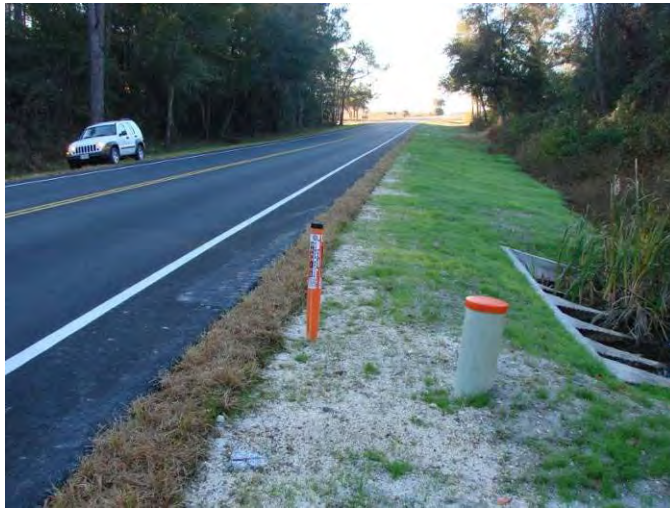
AVENUE B REPAVING PROJECT (DECEMBER 2010)
