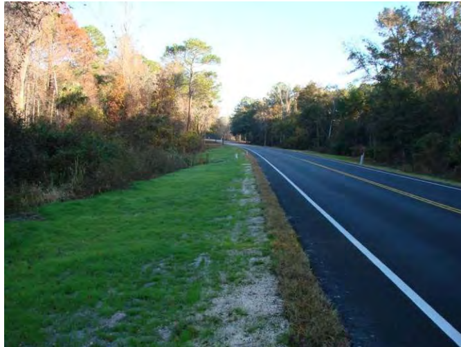
AVENUE B REPAVING PROJECT (DECEMBER 2010)
