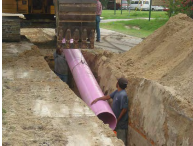
FIGURE 3: CITY OF PALATKA INSTALLATION OF RECLAIMED WATER PIPING
