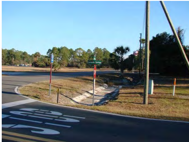
AVENUE C SWALE EXCAVATION AND REPAIR (DECEMBER 2010)
