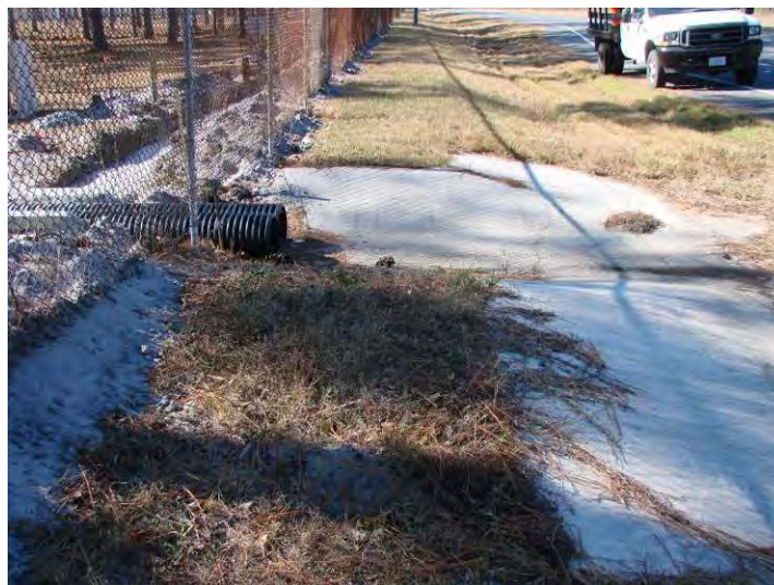
CONSTRUCTION OF NEW DRAINAGE SYSTEM ALONG STATE ROAD WEST 16 (DECEMBER 2010)
