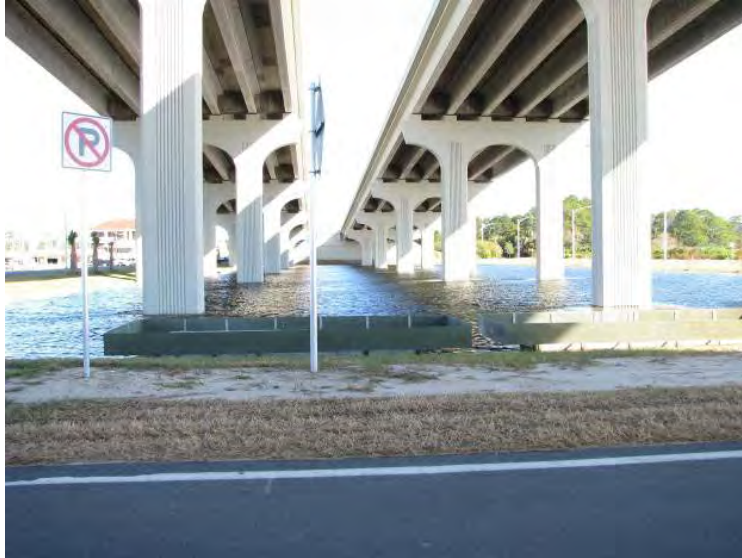
BEACH BOULEVARD STORMWATER RETENTION POND
