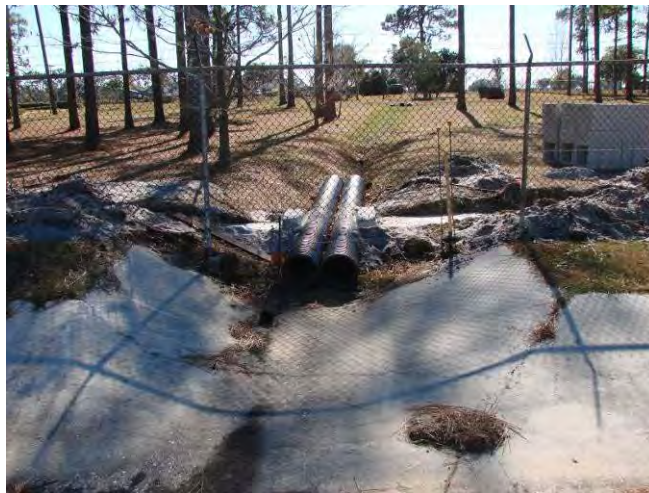
CONSTRUCTION OF NEW DRAINAGE SYSTEM ALONG STATE ROAD WEST 16 (DECEMBER 2010)
