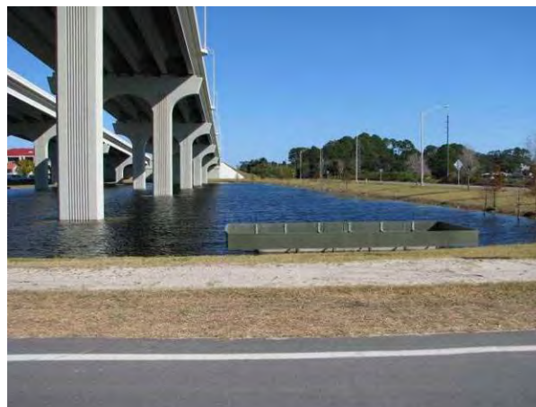
FIGURE 21: BEACH BOULEVARD STORMWATER RETENTION POND IN JACKSONVILLE BEACH
