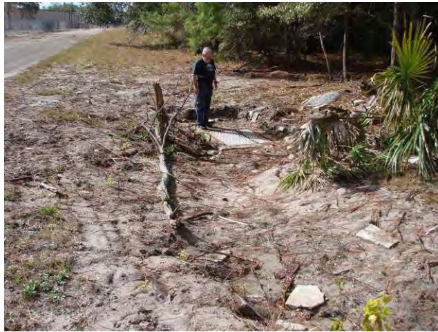
VEGETATION CLEARANCE IN PREPARATION OF NEW SWALE SYSTEM (DECEMBER 2010)
