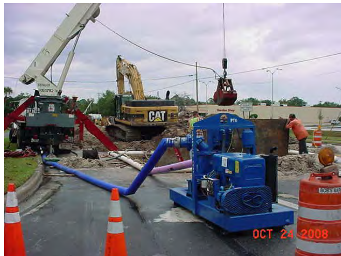
CONSTRUCTION FOR RECLAIMED WATER PIPING
