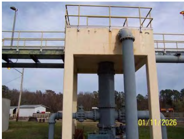
INFLUENT SPLITTER BOX CONSTRUCTED IN 1974
