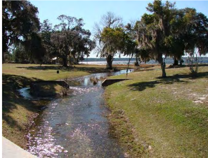
FIGURE 25: CAMP BLANDING KINGSLEY LAKE OUTFALL TO BLACK CREEK
