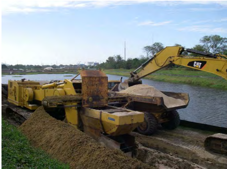
INSTALLATION OF HYDRAULIC BARRIER TRENCH SURROUNDING UPPER DEER CREEK POND EXPANSION USING ONE PASS TRENCHING TECHNOLOGY
