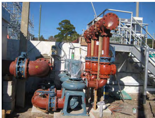
NEPTUNE BEACH WWTF UPGRADE
