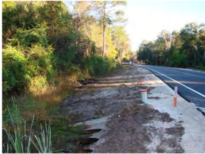
AVENUE B REPAVING PROJECT (OCTOBER 2010)
