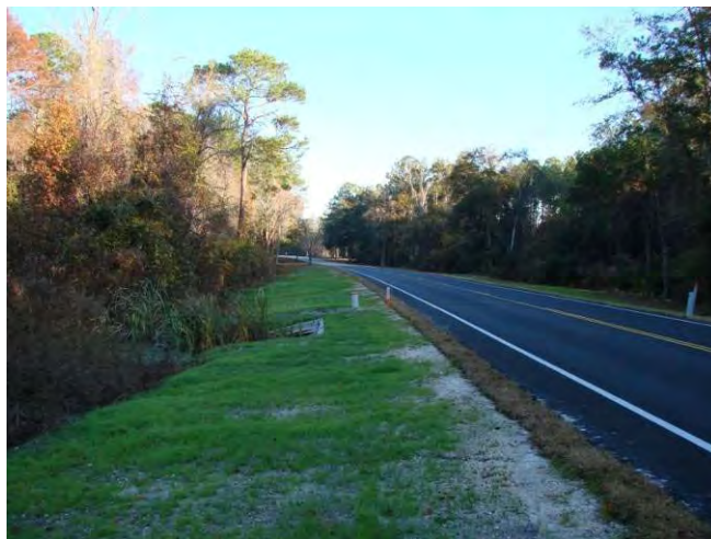
AVENUE B REPAVING PROJECT (DECEMBER 2010)
