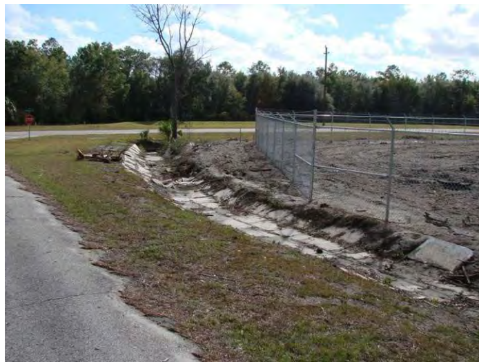
PALMETTO STREET SWALE EXCAVATION AND REPAIR (DECEMBER 2010)
