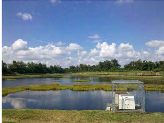
FIGURE 20: COJ INSTALLATION OF MAPS AT THE UPPER DEER CREEK POND EXPANSION
