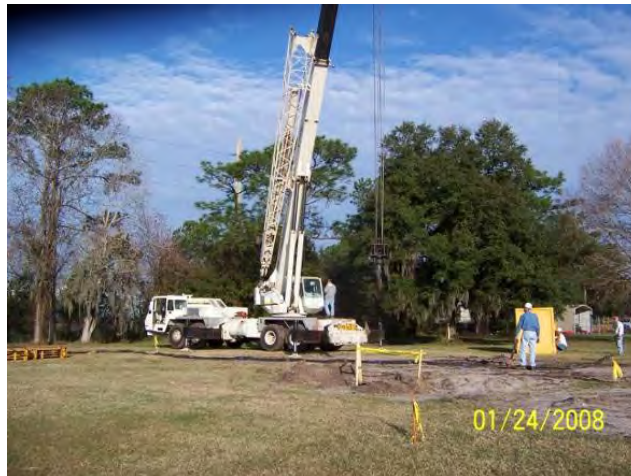
PBM CONSTRUCTORS PREPARING TO DRIVE PILES FOR DIGESTER #2
