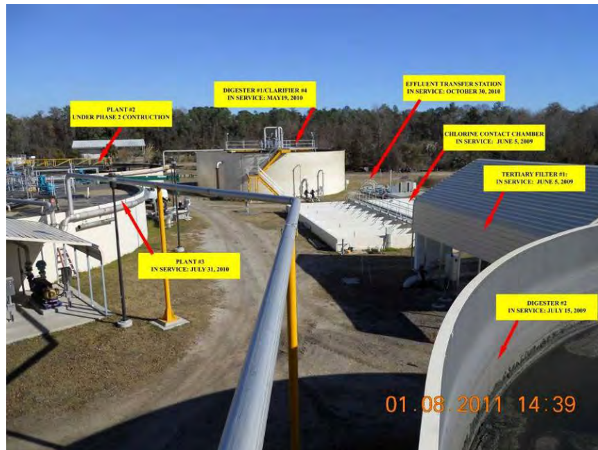
ASH STREET ADVANCED WWTf SITE LOOKING EAST FROM DIGESTER #2
