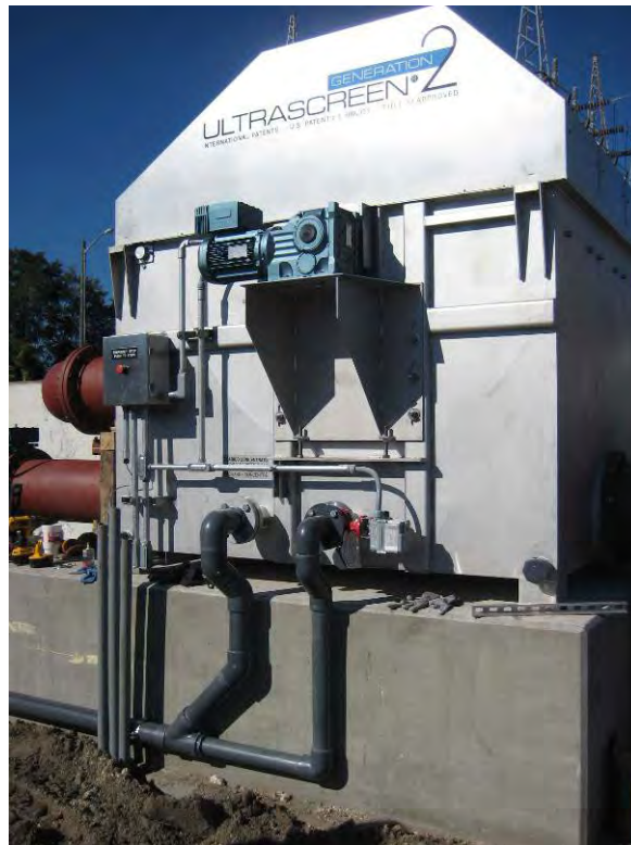
NEPTUNE BEACH WWTF UPGRADE
