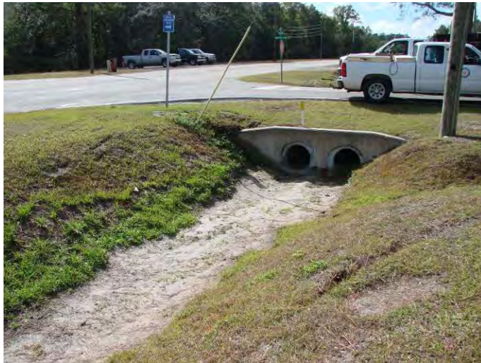
AVENUE D SWALE RECONSTRUCTION WITH NEW CULVERT PIPING (OCTOBER 2010)
