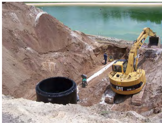
TIE-IN AT THE POND
