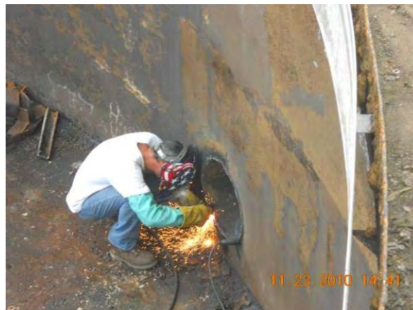
DEMOLITION OF EXISTING INTERNAL PIPING IN PLANT #2
