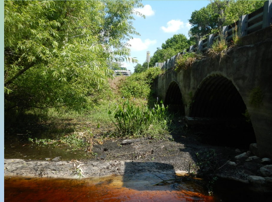
Bridge crossing at Bowlegs Creek. Site is downstream of bridge.
