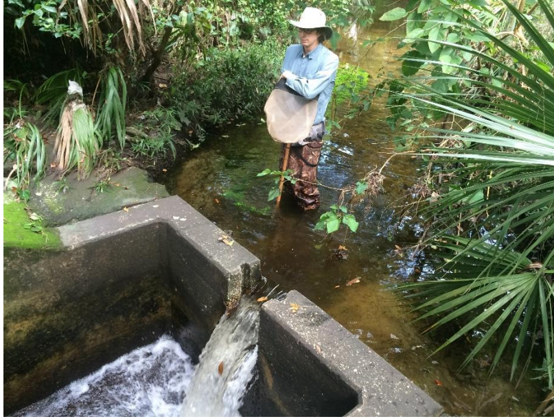
Figure 3-6. Sweetwater Branch upstream of KGS. Note the water control structure modifying natural hydrology.
