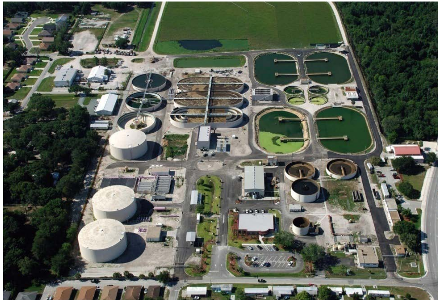
Figure 1. Aerial view of the City of Plant City Water Reclamation Facility.
