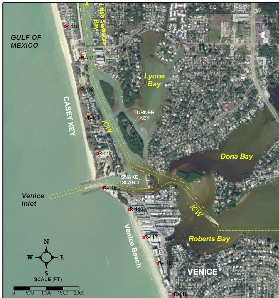
Venice Inlet Aerial Photo (Present conditions)
