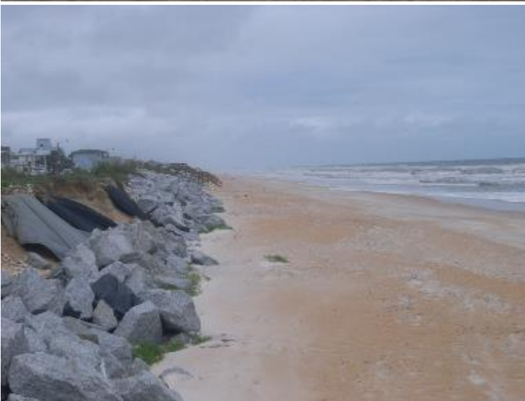
View north R-90; south end of roadside revetment (23 rd St.
