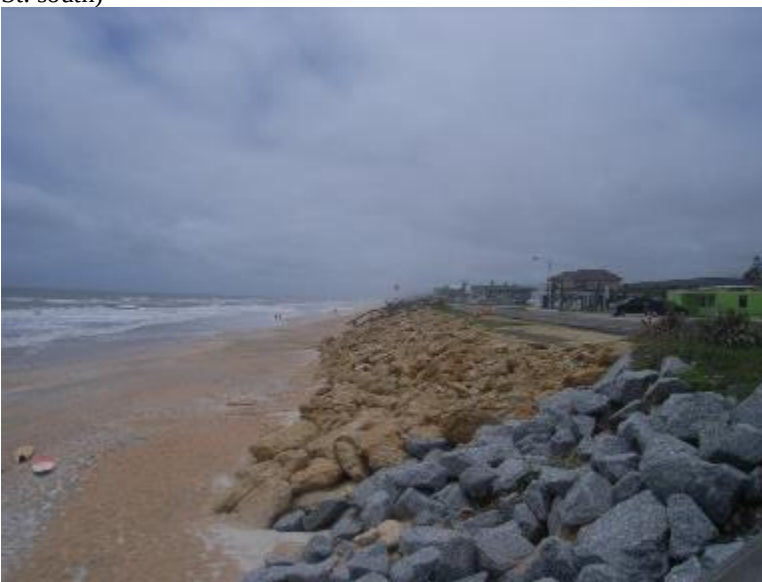
View south from same location showing post storm repairs.
