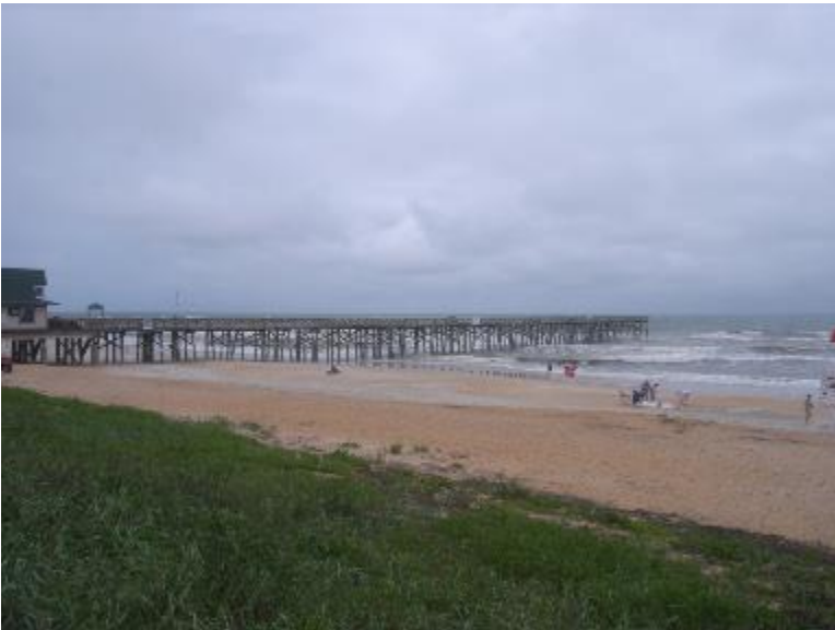
View of south side of Pier.
