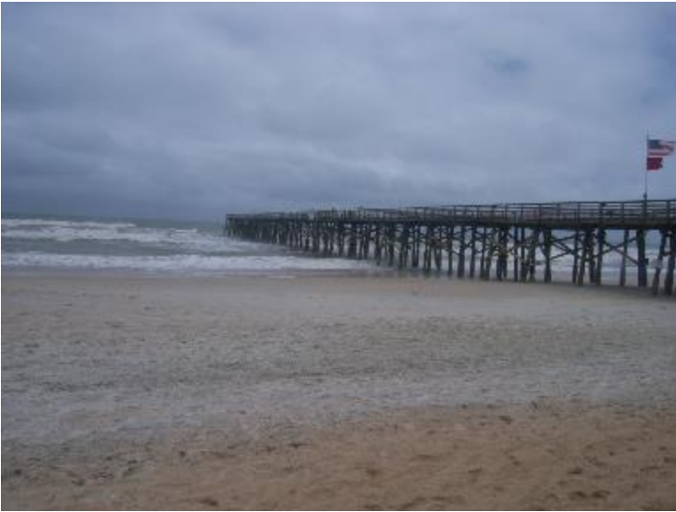
North side of Pier (repairs are still ongoing)
