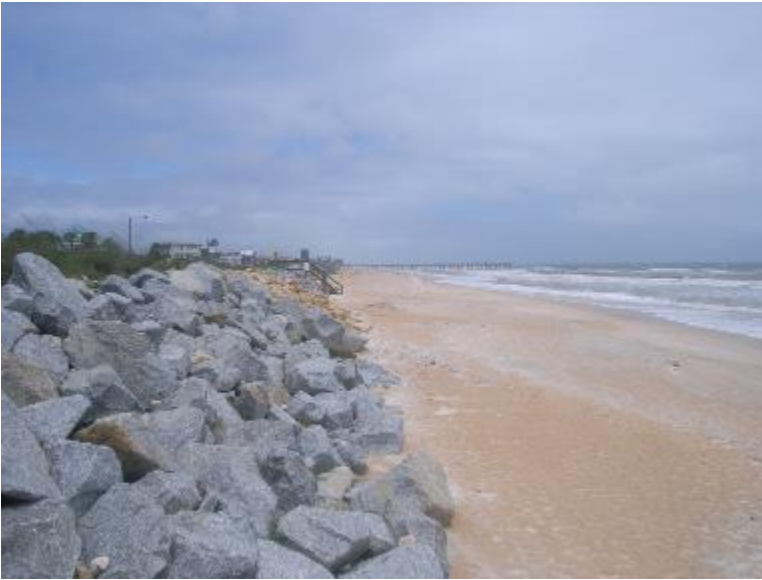
View north from R-81; north end of road side revetment. (11 th
