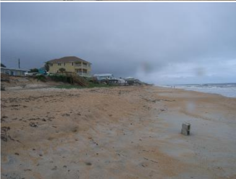
View north from R-57 (south end of future seawall)
