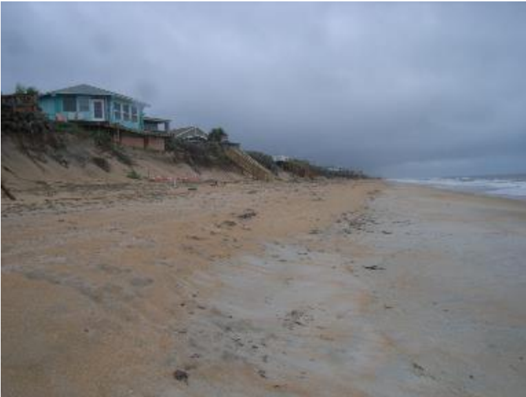
View north at or near R-55.5 (north end of future seawall FL-
