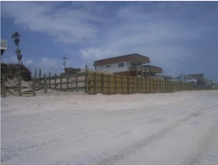
View of south return wall SJ-1311 AR E
