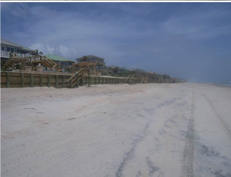
View north at or near R-91 showing existing seawalls.
