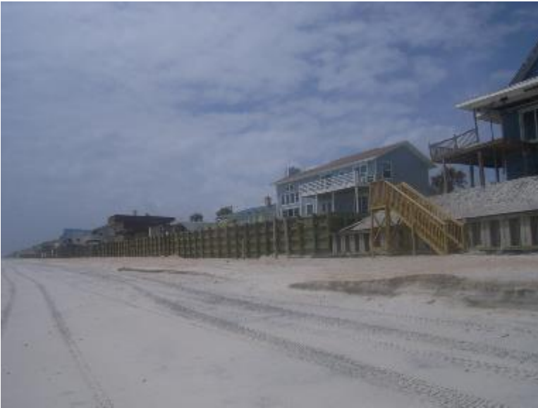
View south from same location (see permit SJ-1311 AR E)
