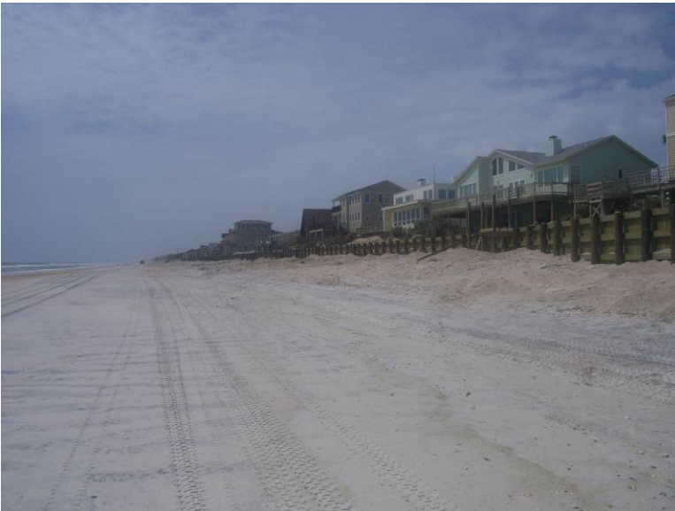
View south from same location showing new wall
