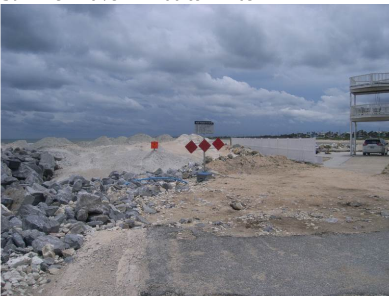
View of street end of Old A1A R-200. Showing fill placed by current dredging project.
