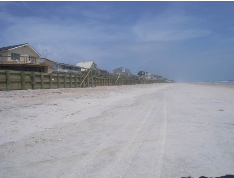
View north of existing seawalls from 2941 SPV Blvd., see SJ-
