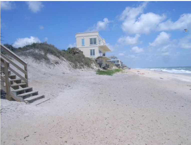
View north from R-113 (SJ County public beach access)
