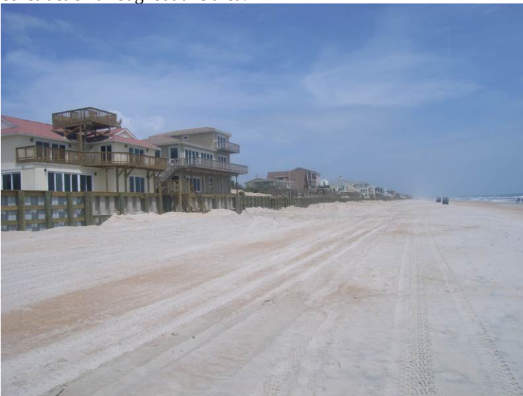
View north at or near R-93 showing new wall construction.
