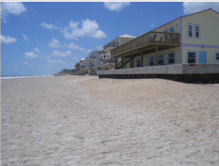
View south from same location to revetment.
