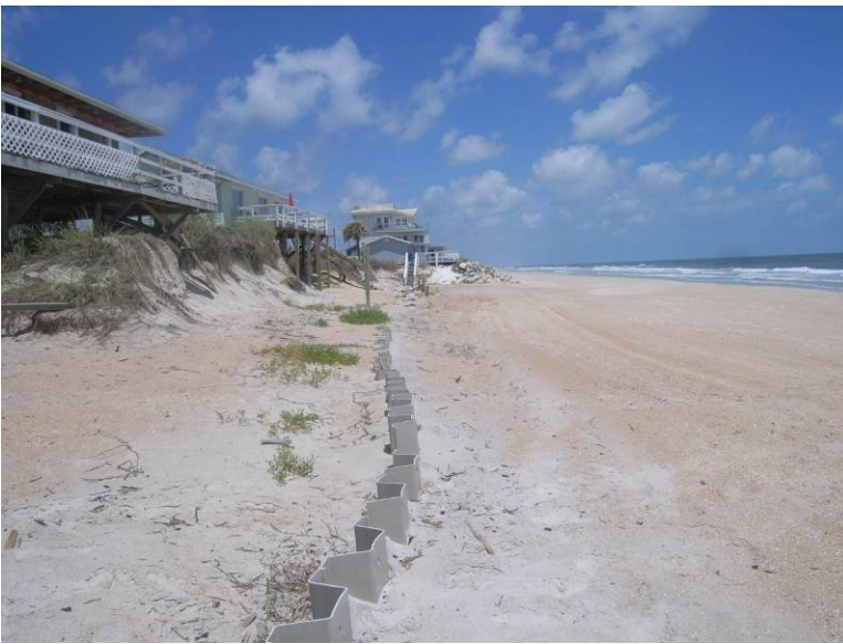
View of south side of revetment.
