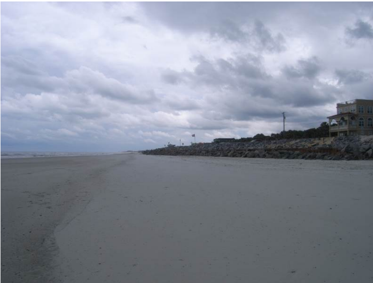
View south of revetment located at or near R-199
