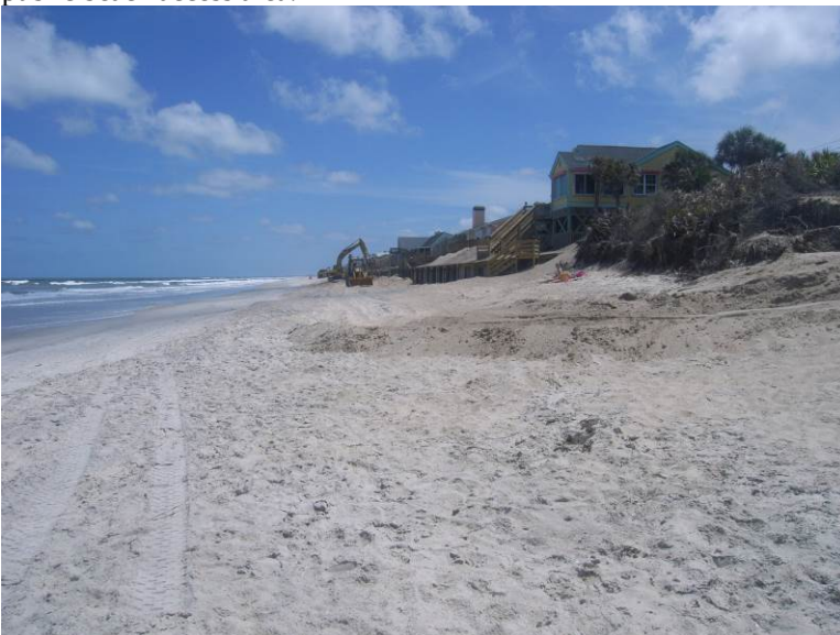
View south of new seawall construction located R-95
