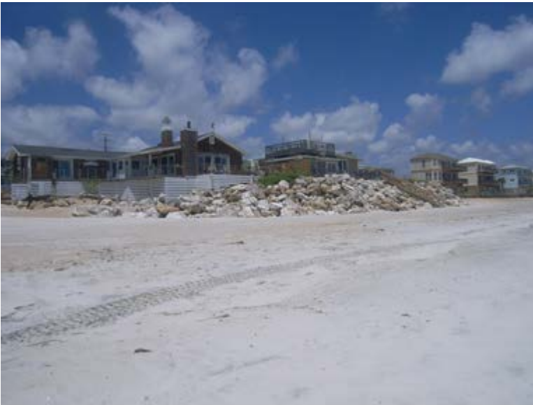
View of revetment.
