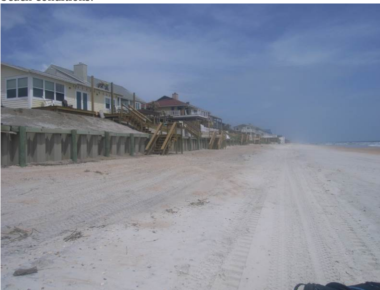
View north at or near R-90 Showing existing seawalls.
