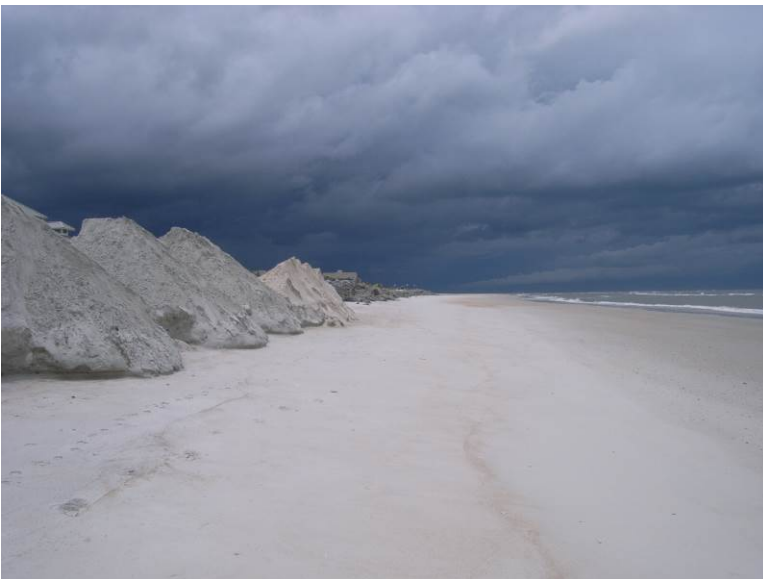
View north from same location to road side revetment.
