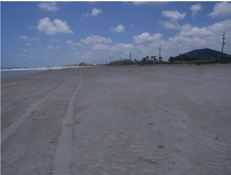
View south from south side of revetment to R-115
