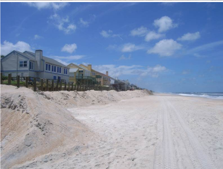
view of new wall construction located just north of R-97
