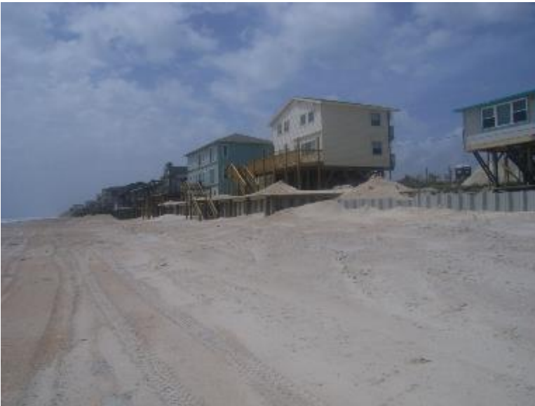
View south of new seawall located 2789 to 2807 SPV Blvd.
