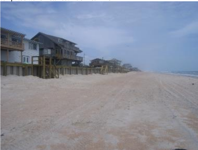
View north just south of R-87 (2801 SPV Blvd.)
