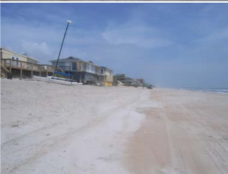
View of properties not installing seawalls located just north of R-94
