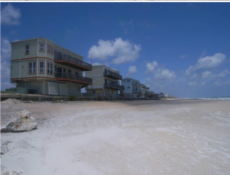
View north from revetment.
