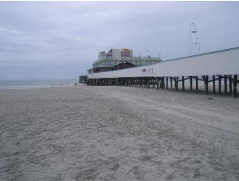
North side of pier
