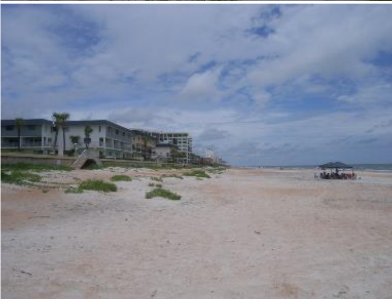
View north at or near R-48.5
