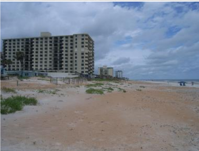
View north at or near R-42
