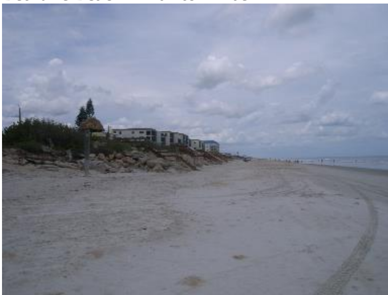
View north at or near R-204.
