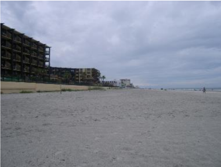
View north at or near R-98.5
