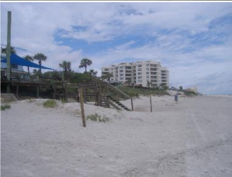
View north at or near R-61.5
