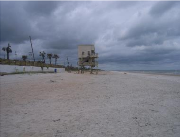
View north public beach access area located T-39.5
