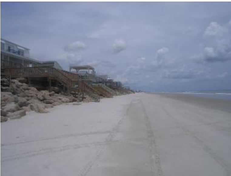
View north at or near R-205
