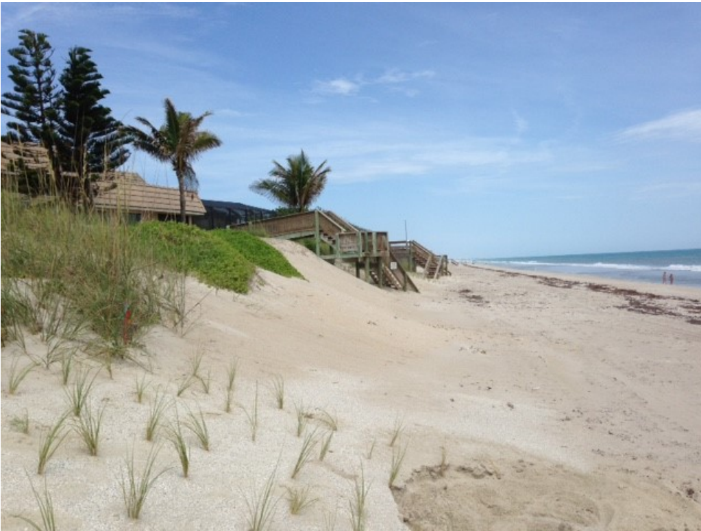
13. View looking north along the beach at ~R-153 toward the 3125 A1A, Melbourne Beach address. There is an existing tube structure at this residence.
