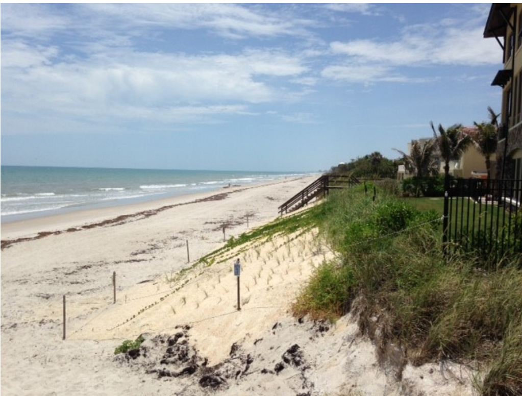
8. View looking south at R-95.5, just seaward of the Desoto access and Ocean St. Pictured here is the north property on Ocean Street where fill was recently placed under the Hurricane Matthew Emergency Order.
