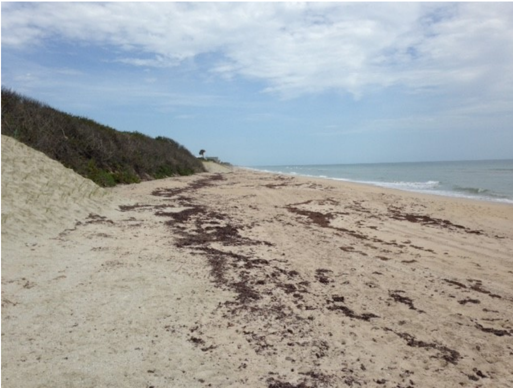
17. View looking north along the beach at ~R-187.5 just north of the Sebastian Beach Inn. As observed in the photo beach compatible fill and supplemental dune plantings were placed here by the county following Hurricane Matthew.
