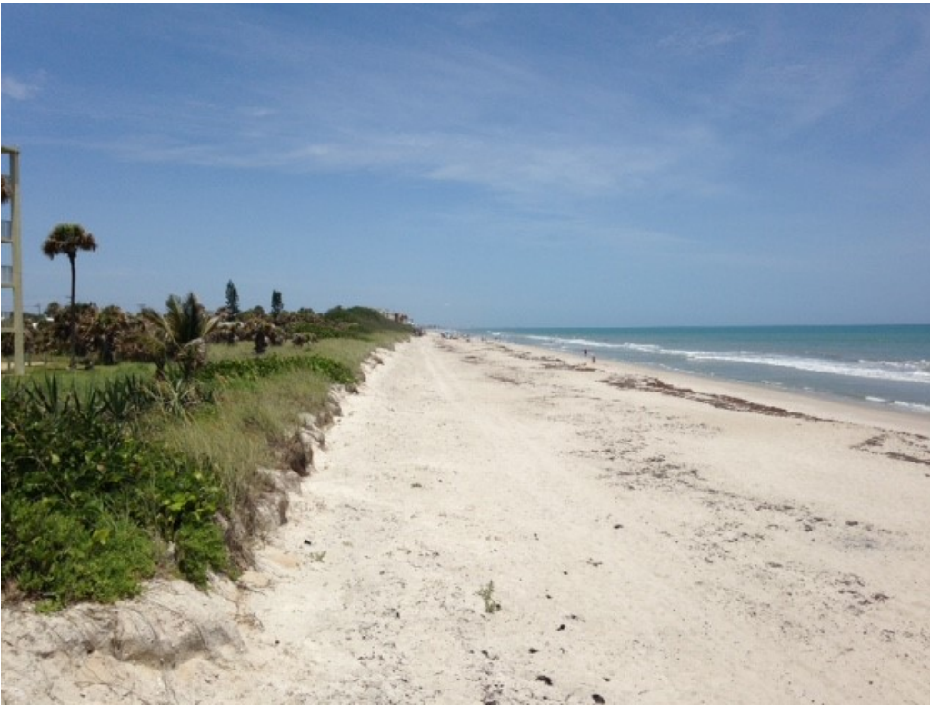
7. View looking north at R-95.5, just seaward of the Desoto access and Ocean St. Pictured here is a 2-4' landward scarp.
