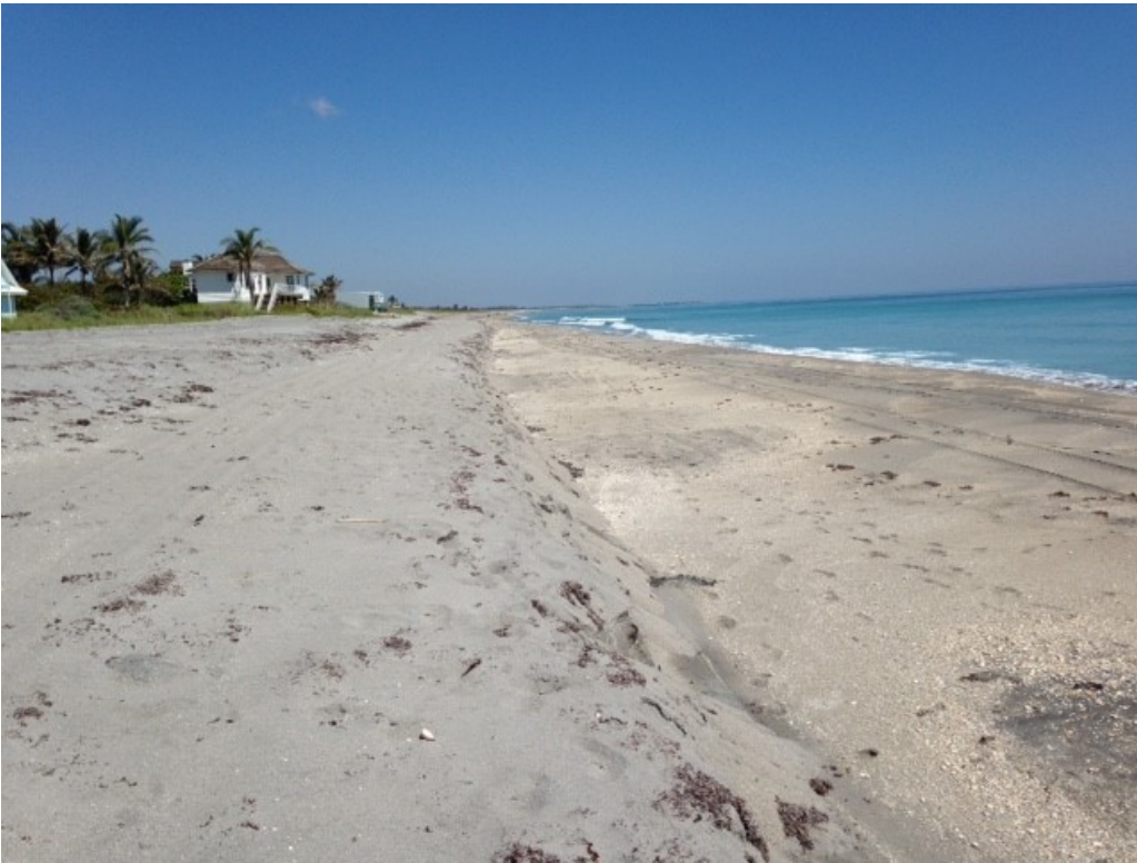
12. View looking north from ~R-78.5 seaward of the 141 N. Beach Rd. area. Prior to 2016, this area was chronically plagued with highwater incursions and steep vertical scarping. However, with the 2016 JCP sand placement project, the beach remains wide. The boundary between the JCP placed sand last year and native beach sand can be seen by the difference in color. This area is currently marked by a 1-3' scarp (pictured). No current problems were noted.
