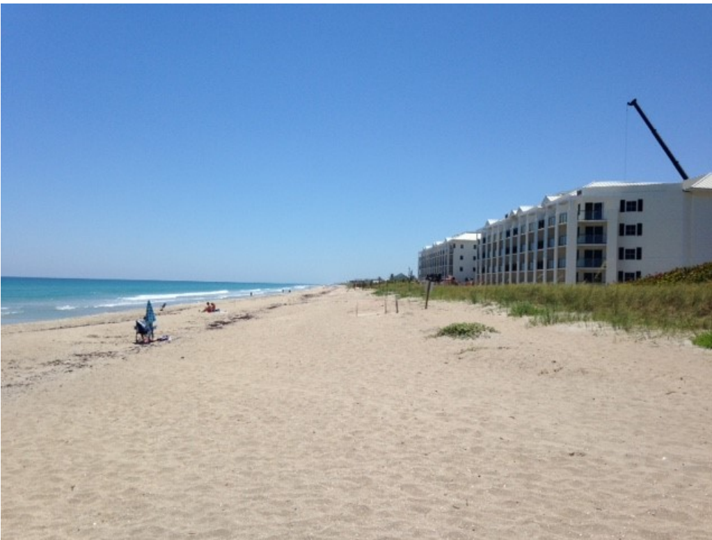
2. View looking south from ~R-5.5 at Jensen Beach Park. Currently the beach is wide with no problem areas noted. As pictured, there are minor amounts of hummocky foredune features trying to establish.
