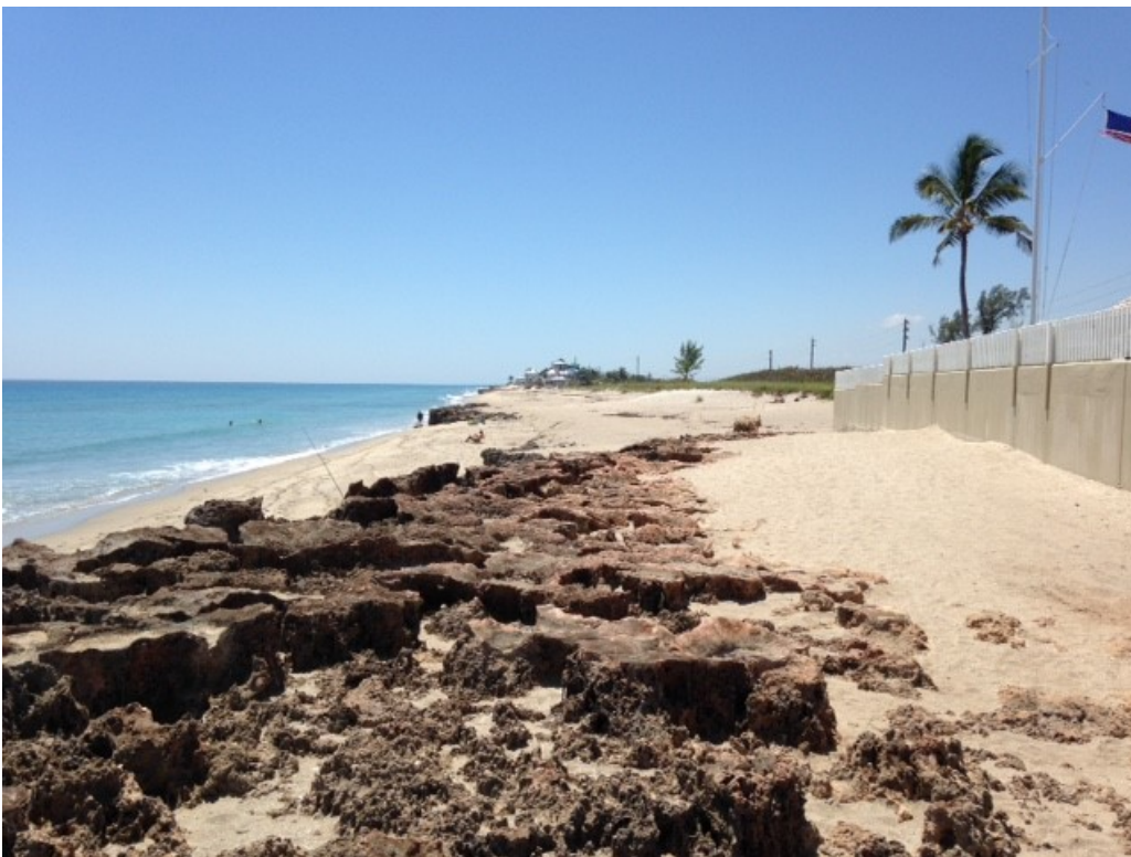
6. View looking south from ~R-29.5 at the House of Refuge. No problem areas were noted.
