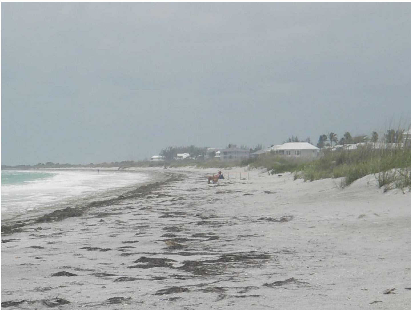
Typical Condition I around R-33. Looking north.
