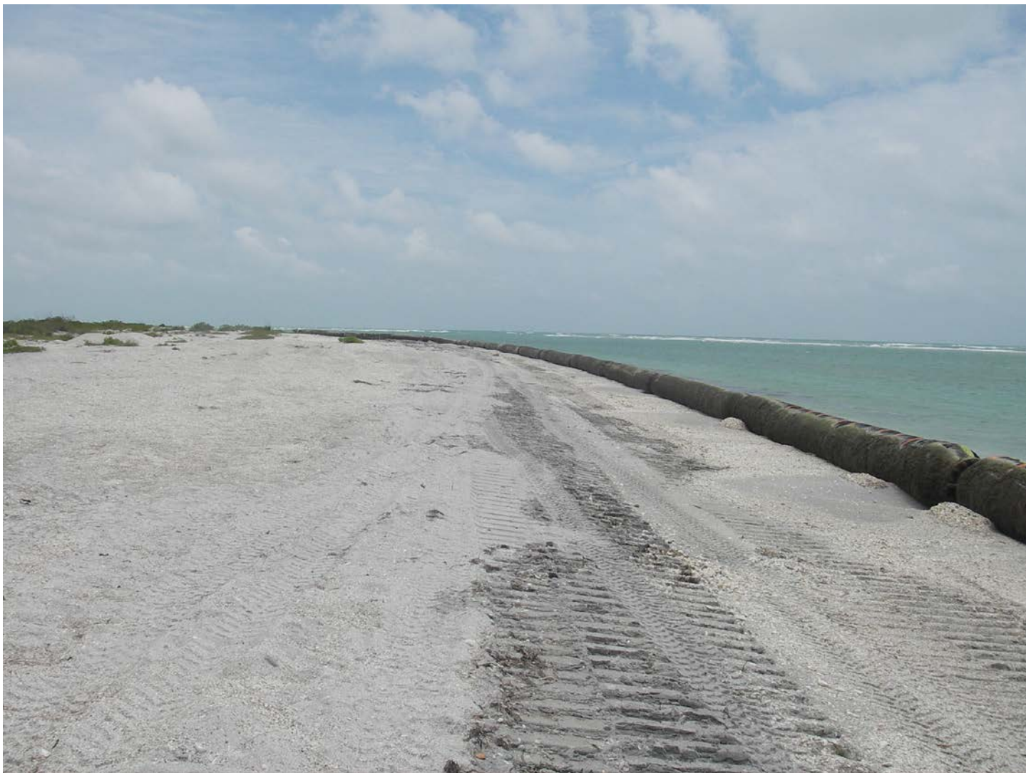
Knight Island side of Stump Pass dredging operation ongoing. Looking southwest.
