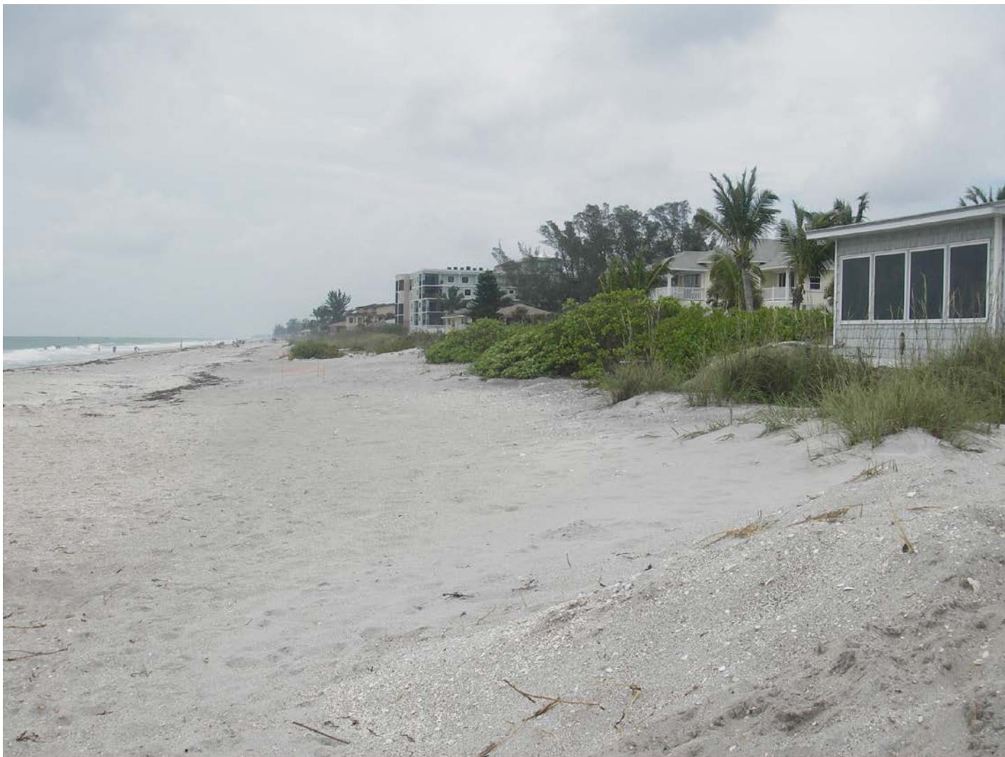
Typical condition for R-12 to 15 is condition I. This is at Wilhelm.
