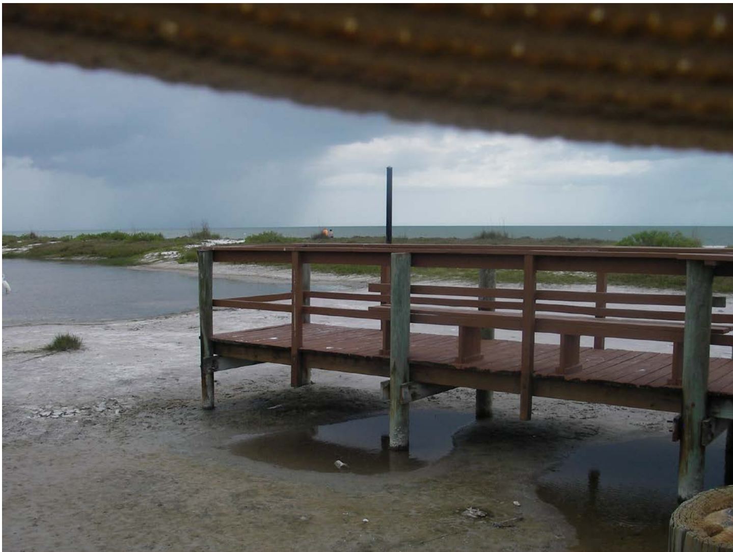
Pier at Caribbean Beach Club 7600 Estero in the CWA lagoon east of R-205.
