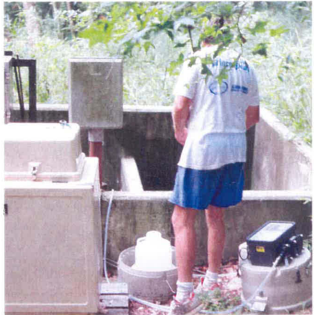
Plant Scholz Ash Pond Discharge – Station PSAP
