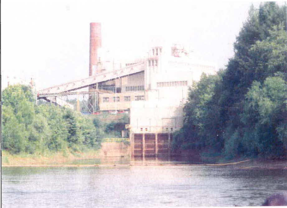
Plant Scholz Intake Canal
