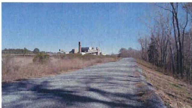
Southern Access Road Facing NE
