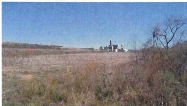
SW Access Road facing NE
