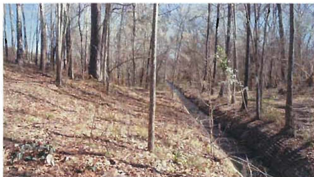
Base of Berm with Outfall
