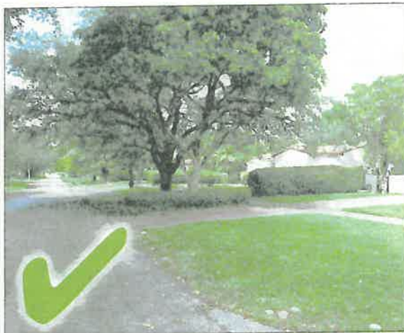
A properly maintained swale. Note that only the driveway approach is paved.
