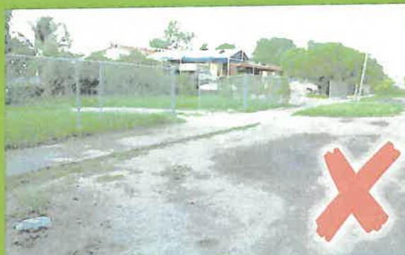
Note evidence of cars parking on the swale and the compacted soil.
