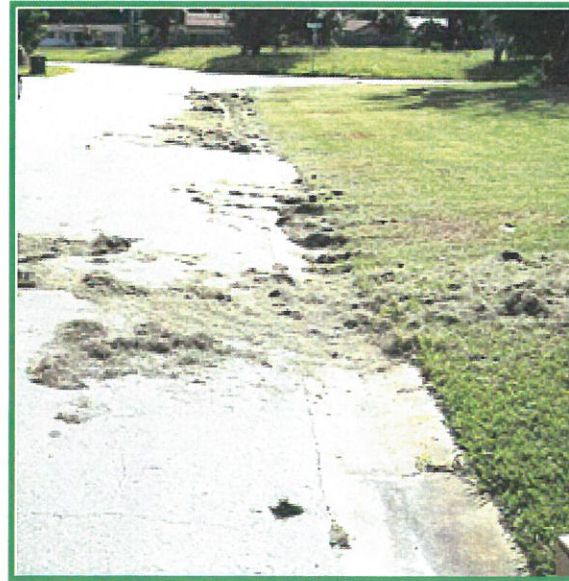
▲ Violation of local, state, and federal laws.
