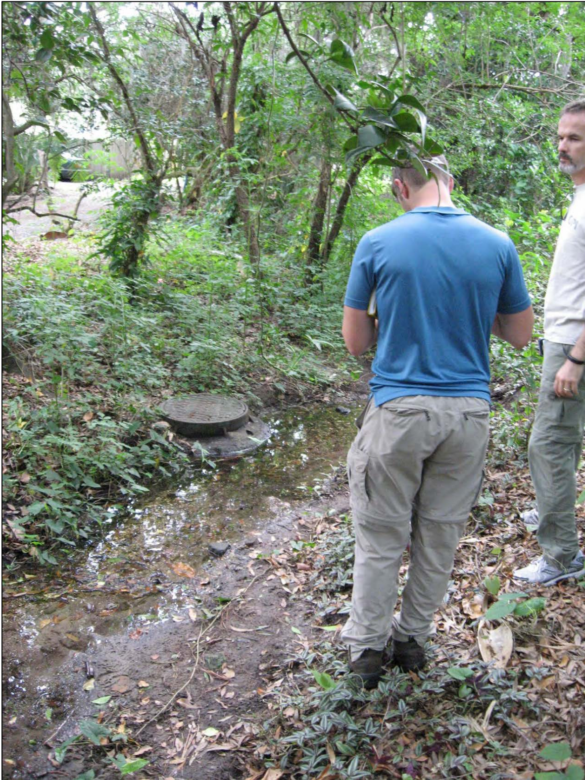
Figure 13. Site M – Sanitary sewer line adjacent to surface water conveyance feature.
