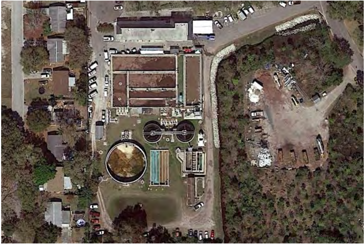
Figure 15. Site O1 – the On Top of the World wastewater treatment plant. Note the rip rap rubble along the banks of Channel C of Alligator Creek, adjacent to the plant.
