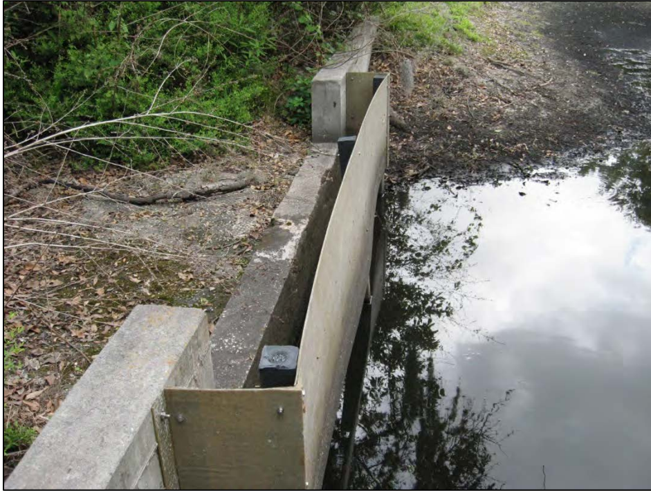
Figure 26. Site N – Coachman Reserve - Stormwater outfall structure from townhome community.
