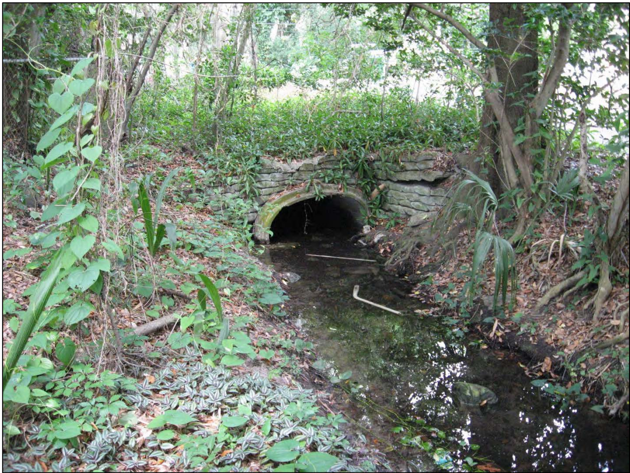
Figure 22. Site M – Surface water ditch adjacent to sanitary sewer pipe and manhole.
