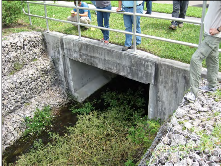
Figure 30. Site P – Coachman Ridge – Gabion system at the headwall along the Wetherington Road crossing of Alligator Creek.
