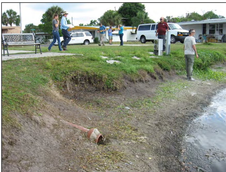
Figure 11. Site C – Boulevard Estates Mobile Home Park – Pond margin with pet and bird feces, as well as numerous pipes. A sewage odor was detected at the pond.
