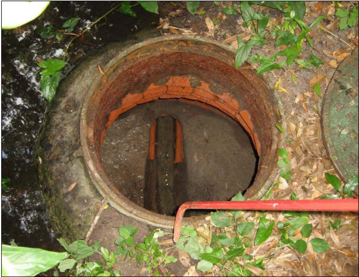
Figure 24. Site M – Manhole in sanitary sewer line adjacent to surface water conveyance feature.
