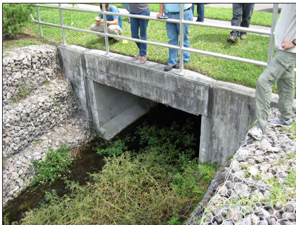
Figure 17. Site P – Coachman Ridge – Gabion system at the headwall along the Wetherington Road crossing of Alligator Creek.
