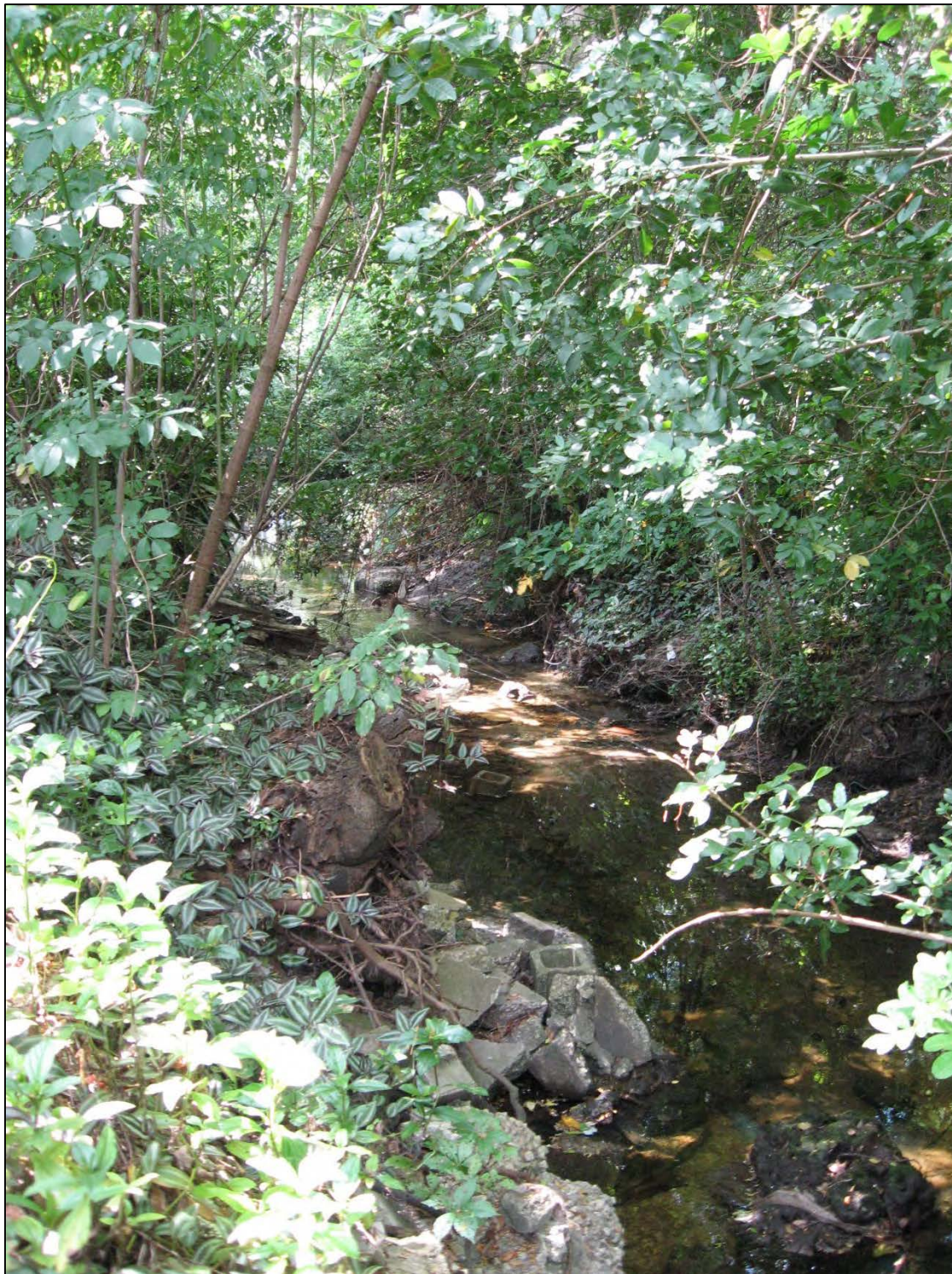
Figure 16. Site F – Alcove Park Mobile Home Park - Deeply incised banks of Channel C of Alligator Creek.
