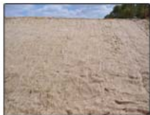
Apply the powder to the group either dry or with a hydroseeder, cover with matting on steep slopes.
