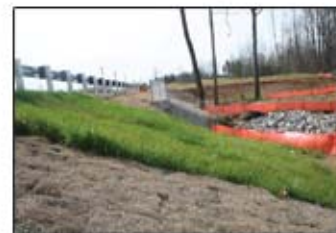
Despite the steepness of the slope the seed was able to germinate and the soil is no longer bare. The erosion has been stopped.
