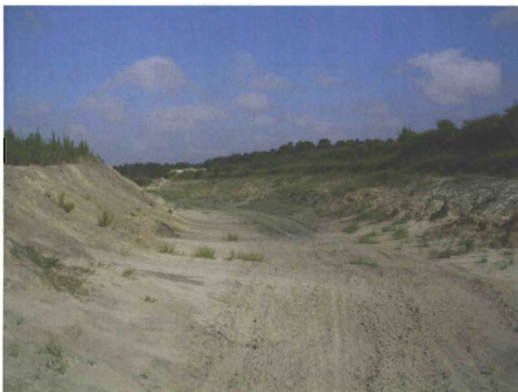
Berm and recharge ditch in northern portion of property, looking west.
