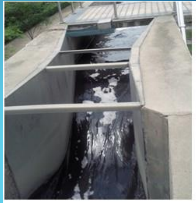
Pre-built metal Parshall Flume installed in a medium size canal
