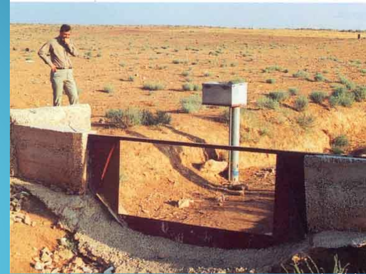
Metal plate Rectangular Weir installed in an earthen channel
