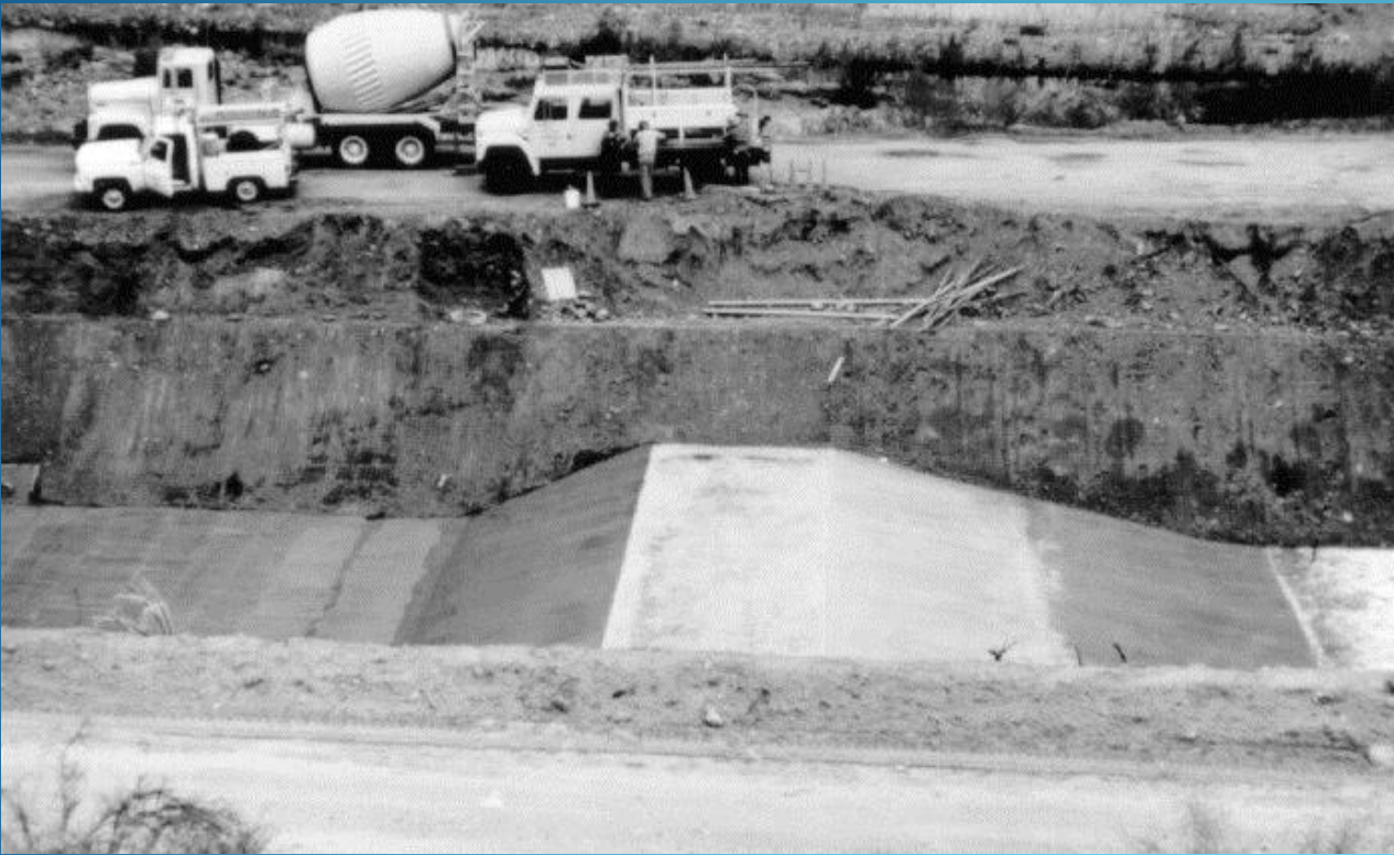
Concrete Long-throated Flume being built in a large capacity stream. Critical depth develops on the broad-crested weir section
