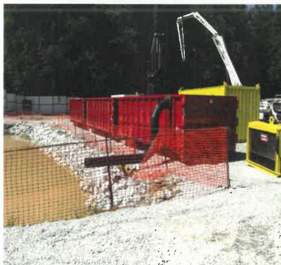
Three tanks make up the system and involve the use of Floc Logs and particle curtains to treat incoming water and remove sediments before discharge.
