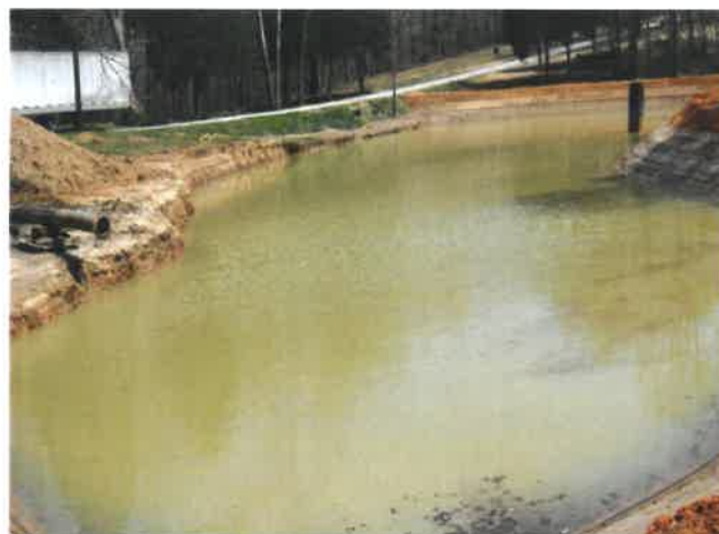
The dredge spoils discharged into the stilling pond through the pipe on the left and discharged through the riser pipe on the right.
