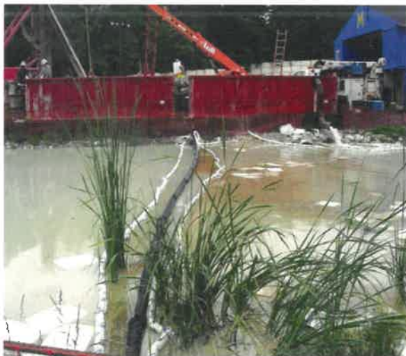
Three tanks make up the system and involve the use of Floc Logs and particle curtains to treat incoming water and remove sediments before discharge.
