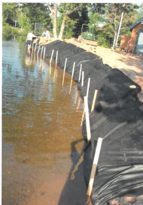
The photo to the left shows the geosynthetic fabric laid on the bank and the sand beginning to be deposited. The photo to the right shows the excess fabric being pulled over the sand and fortified with rock, forming a containment for the sediment.
