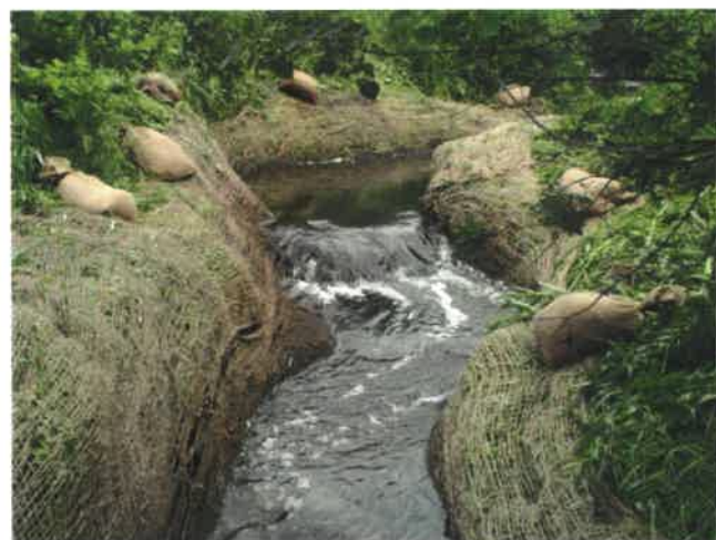
Below: Jute matting was installed along the stream bed and banks.
