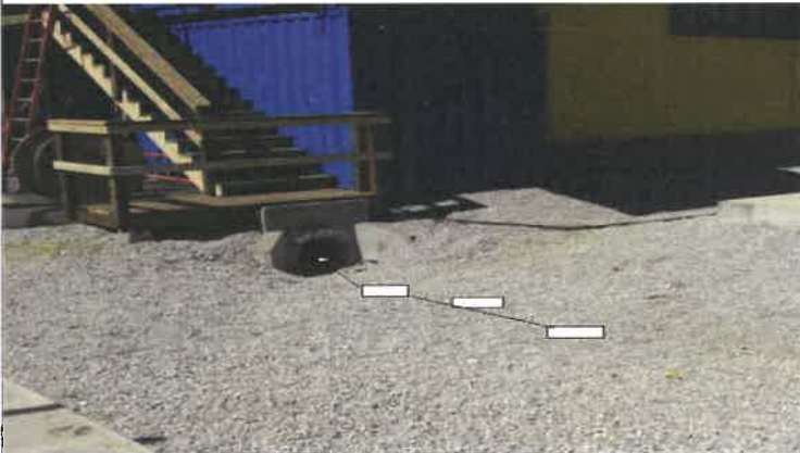
Above: Particle curtain strategically placed to catch the particles that did not settle out by gravity.
