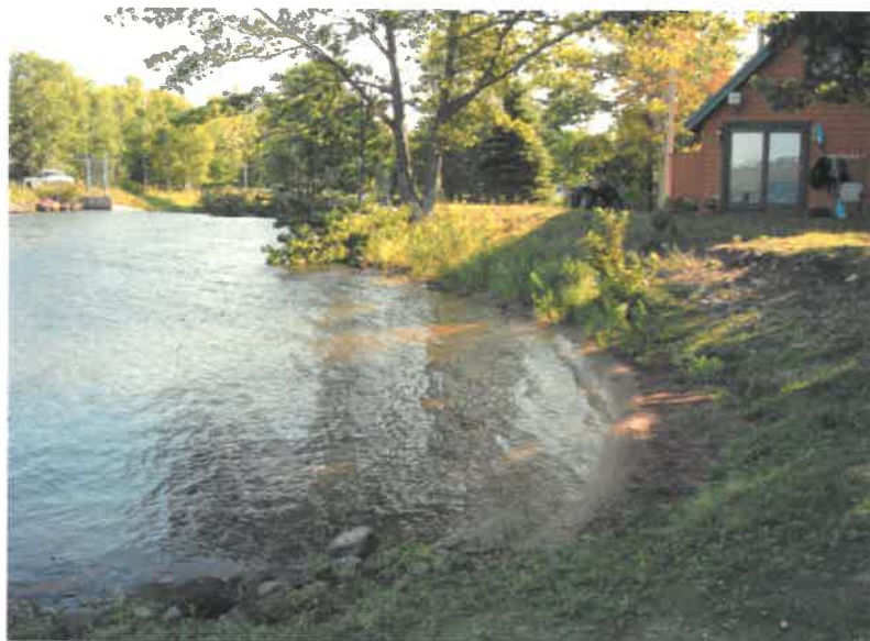
Erosion of the shoreline is clearly visible in the bank along the right side of this photograph. The dam is seen on the upper left-hand corner of the photo.
