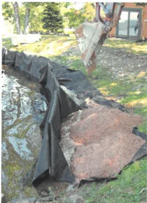
The photo to the left shows the geosynthetic fabric laid on the bank and the sand beginning to be deposited. The photo to the right shows the excess fabric being pulled over the sand and fortified with rock, forming a containment for the sediment.
