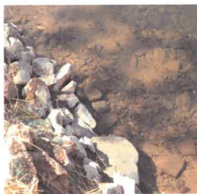
Left: Completed bank structure consisting of sand, rock, and top soil.
