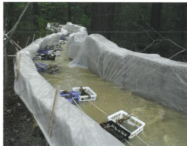
The soil-specific Floc Logs were secured into plastic crates in the mixing/reaction portion of the treatment system where the polymer would react with suspended sediment.
