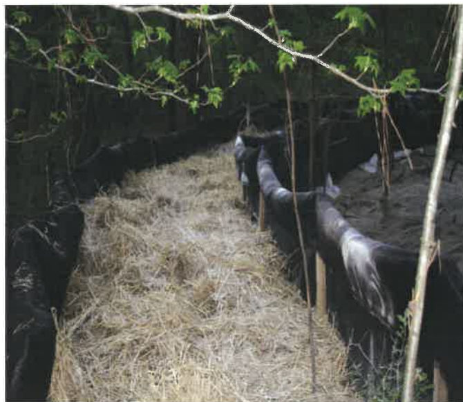
The treated water passed across the jute dispersion field before passing through the sediment retention barrier filled with straw and polymer where final polishing occurred.
