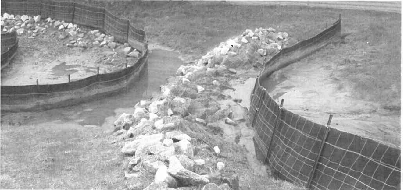
Particle attachment to jute matting with polymer after rain event
