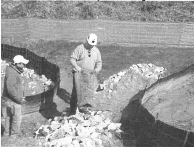
Cover rock check with jute matting
