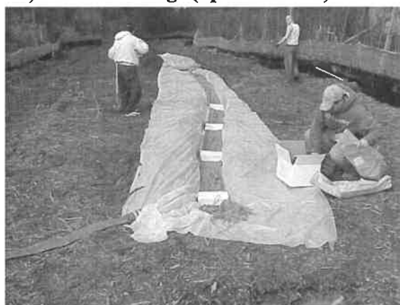
4) Place Floc Logs (upstream end)
