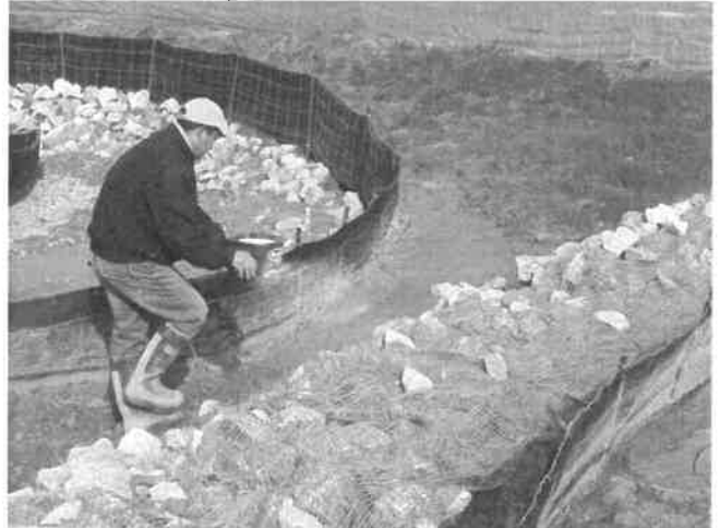
Apply Silt Stop powder over rock check
