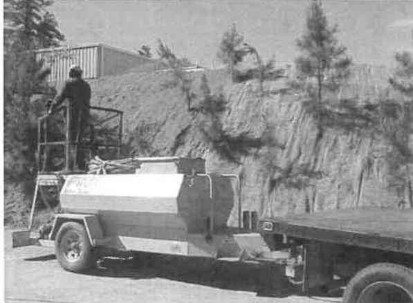
5) Spray onto slope
