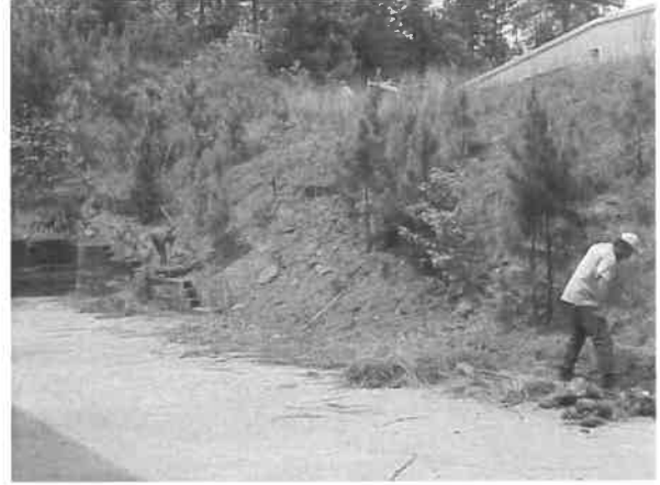
2) Fill rills and gullies
