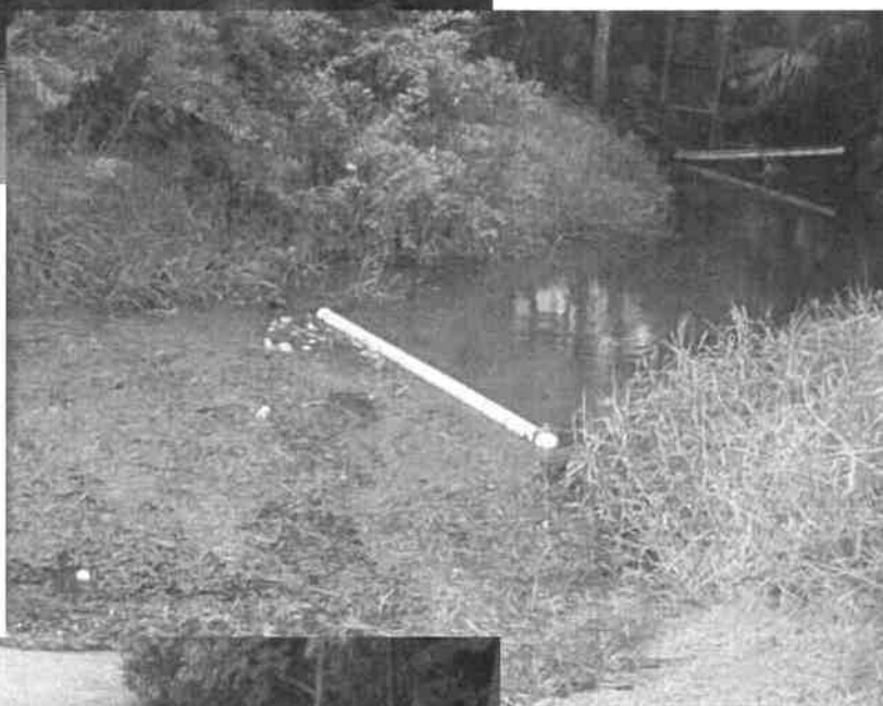
(Right) The particle curtain floating in the stream. Note the other particle curtains in place further down stream in the background.
