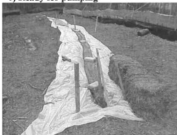
6) Ready for pumping
