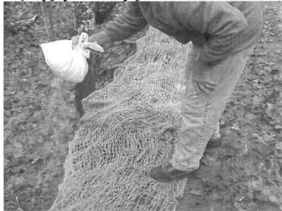
4) Apply Silt Stop powder
