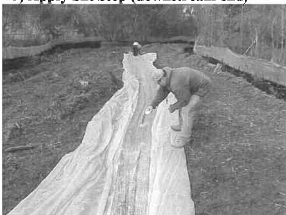
5) Apply Silt Stop (downstream end)
