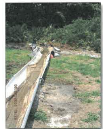
Figure 21. Split pipe with soft matting
