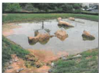
Figure 41. Same pond after BMPs were installed
