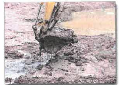
Figure 36. Removing stiffened sediment from a sediment basin
