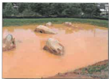
Figure 40. Sediment pond before BMPs were installed
