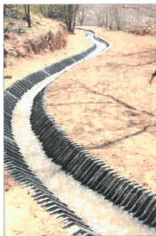
Figure 18. In-ground treatment ditch
