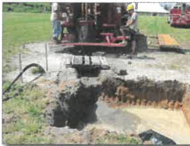
Figure 7. Drilling rig and settling pit
