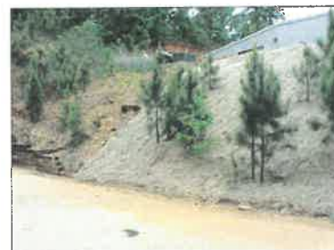
Figure 4. Slope covered with floc collection matting
