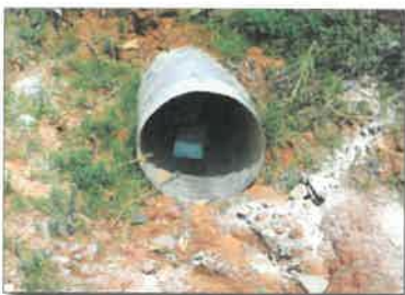
Figure 39. Polymer block in a construction site culvert
