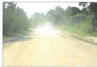
Figure 12. Road dust before applying polymer flocculant
