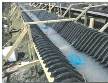
Figure 17. HDPE treatment ditch liner
