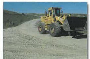
Figure 13. Road dust after applying polymer flocculant
