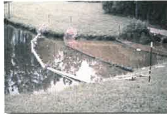
Figure 30. Particle curtains clarifying the input to a pond
