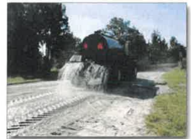
Figure 11. Water truck applying dissolved polymer flocculant
