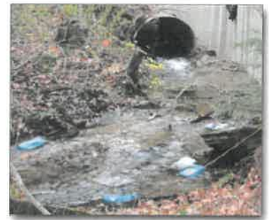
Figure 25. Six of the polymer blocks placed downstream
