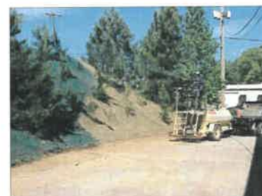
Figure 5. Hydroseeding the slope
