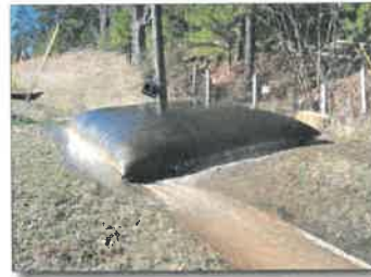
Figure 34. Sediment bag and its treatment ditch
