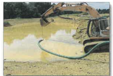
Figure 14. Sediment basin to be dewatered
