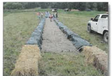
Figure 15. Lower portion of the treatment ditch
