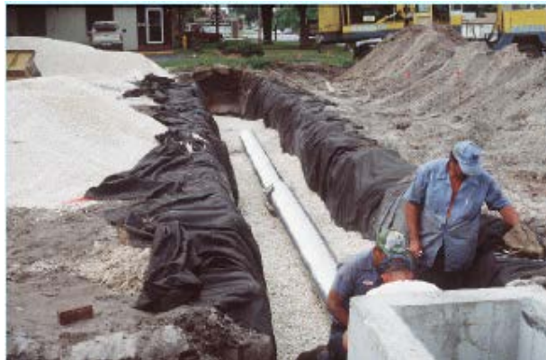
Underground Exfiltration Trenches
