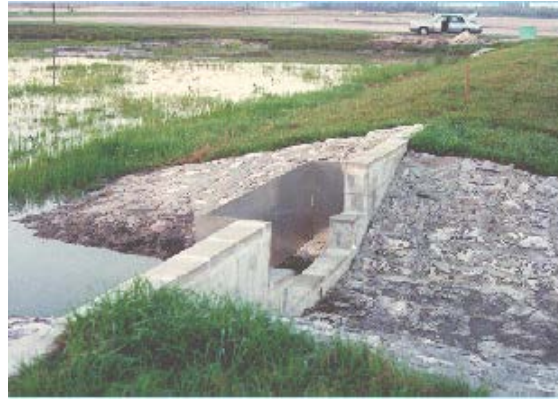
“Wet” Detention Ponds
