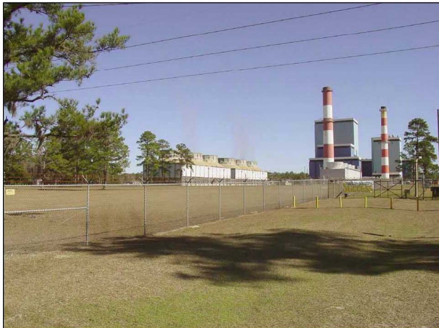
Figure 4.1.4-4 Existing View from Geddie Road Main Entrance Road
