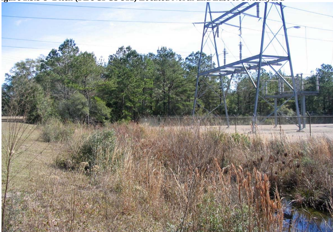
Figure 2.3.5-5 Ditch (FLUCFCS 511) Located North and East of Switchyard
