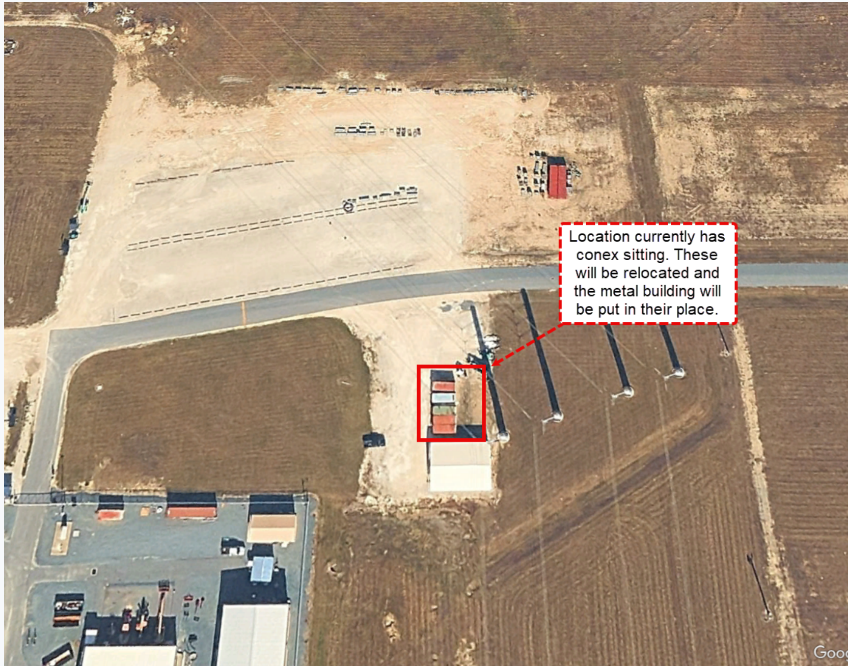
Close-up submitted exhibit showing the existing Connex units and project location.
