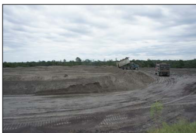
Fly Ash Placement
