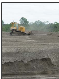
Spreading Fly Ash
