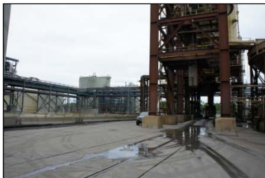
Unit 4 Bottom Ash Silos
