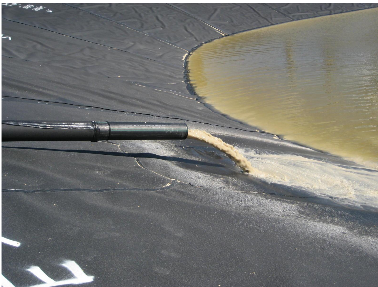
Photograph 1 – Discharge Pipe in Northwest Corner of Back-up Pond (March 4, 2010)
