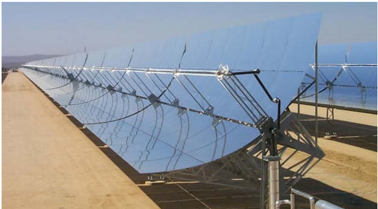
Solar Panels at Kramer Junction SEGS Project
