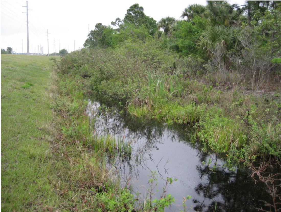
Photo 3. Drainage ditch (FLUCFCS 511) adjacent to Martin Plant access road
