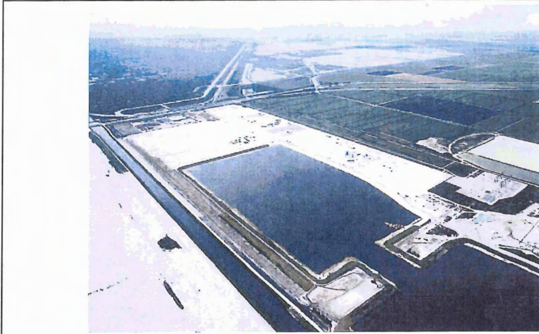
Figure 2.1.0-4. WCEC Site showing Units 1 and 2 under construction. View from northeast to southwest.
