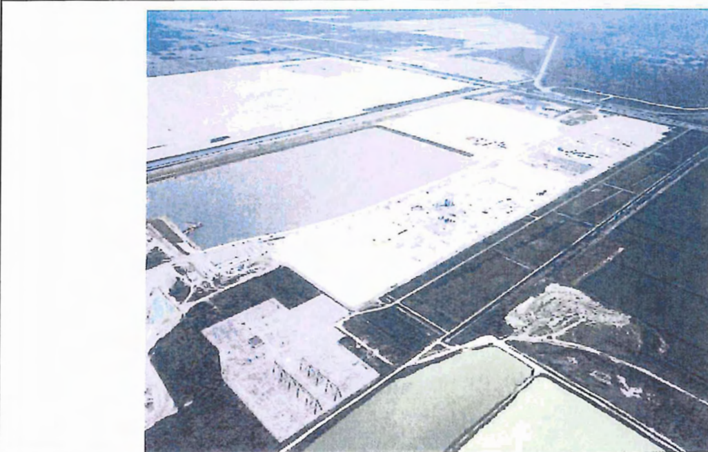
Figure 2.1.0-5. WCEC Site showing Units 1 and 2 under construction. View from northwest to southeast.
