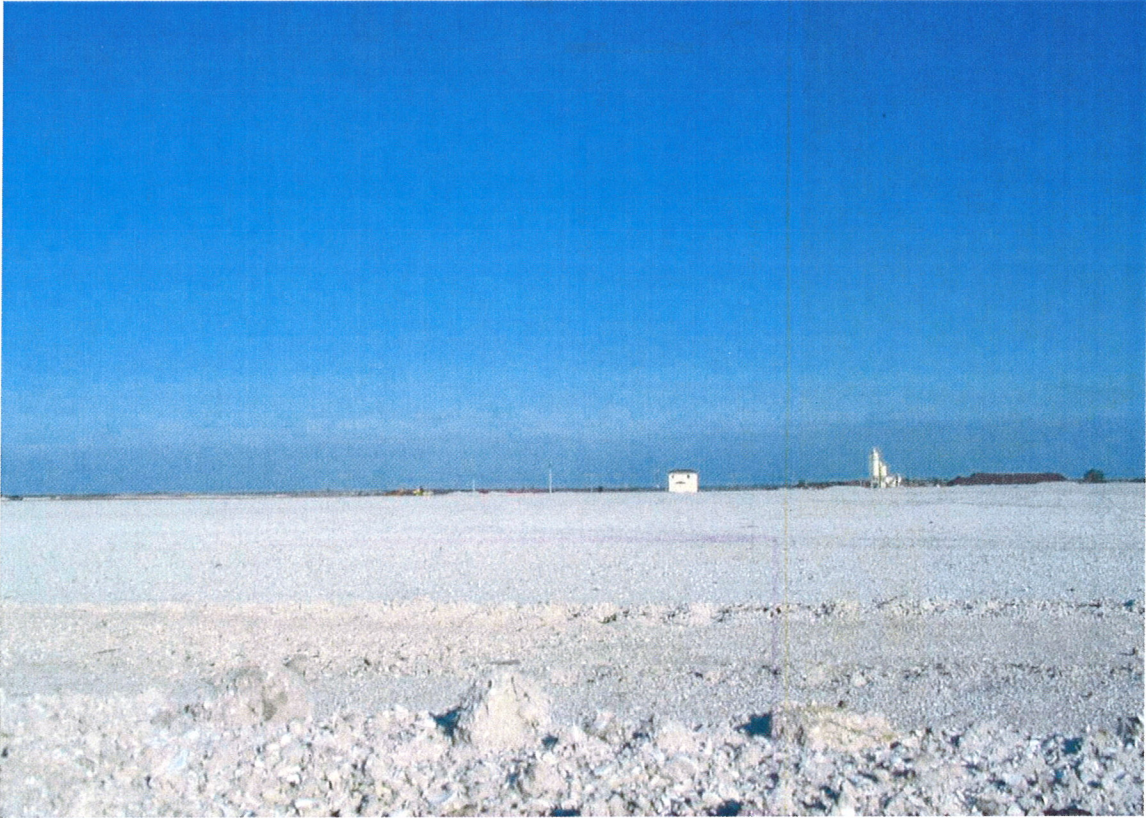
Photo 1. Project Site – open land (FLUCFCS 190) cleared of vegetation, filled, and graded.
