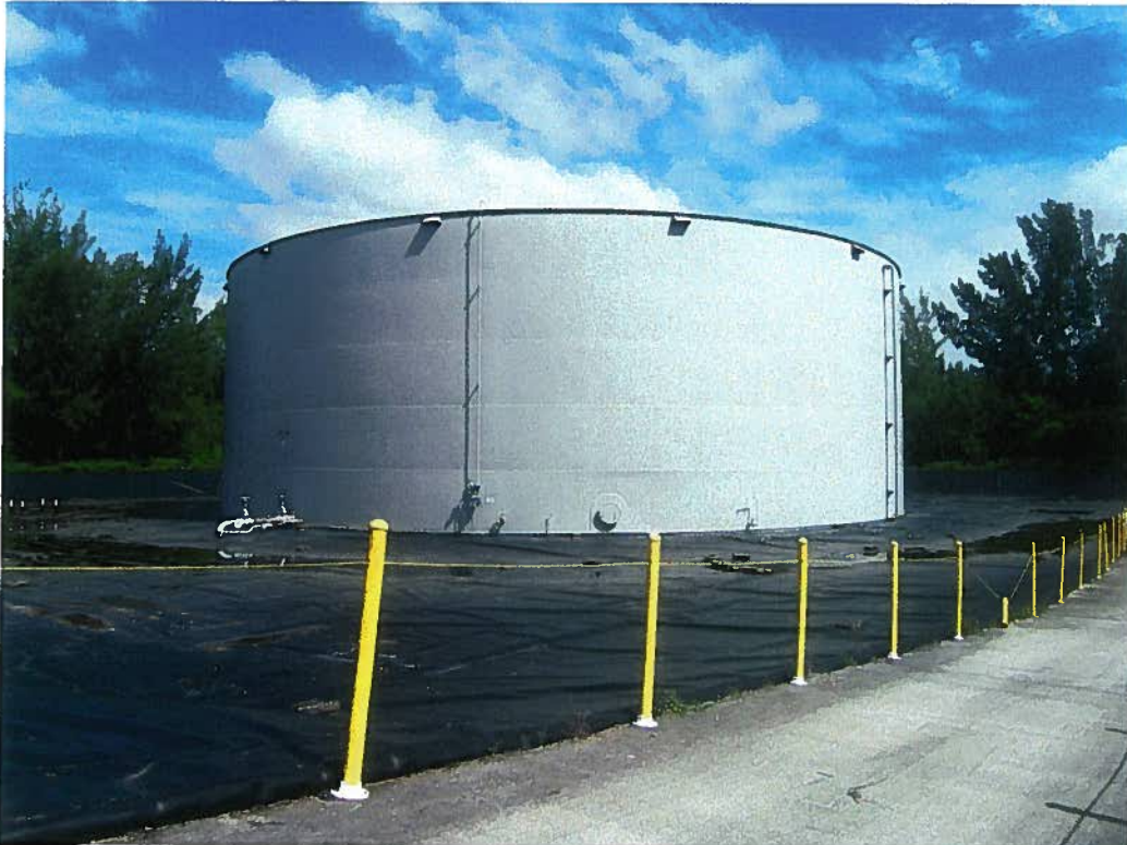
Figure 7. View northeast of Tank 5.
