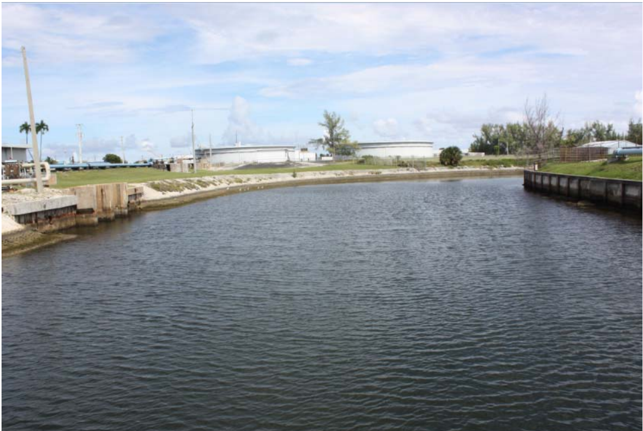
Figure 10.7.1-2. View of discharge canal from Plant
