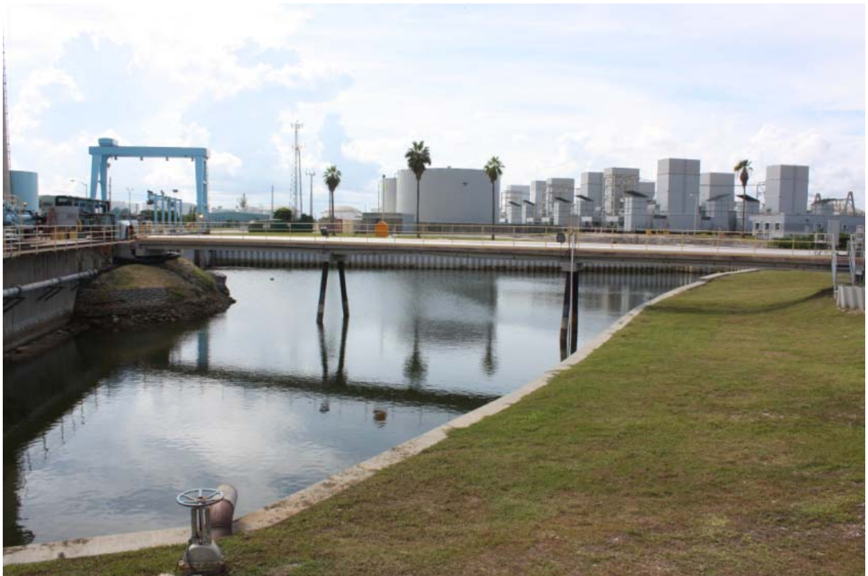
Figure 10.7.1-6. Intake structure and canal near Plant
