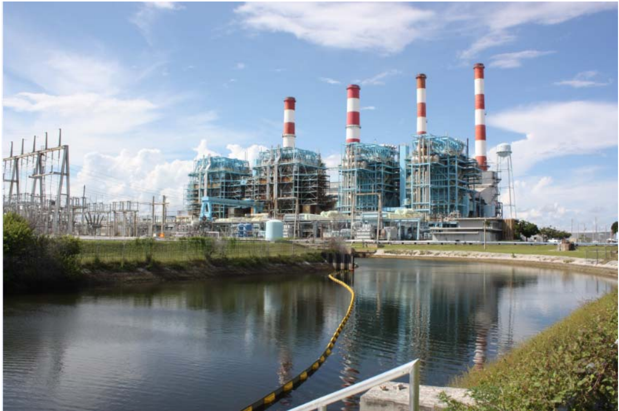
Figure 10.7.1-1. Port Everglades Plant Units 1 through 4 and discharge canal
