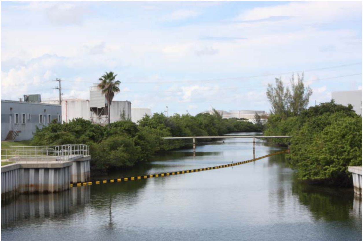
Figure 10.7.1-5. View of intake canal from Plant
