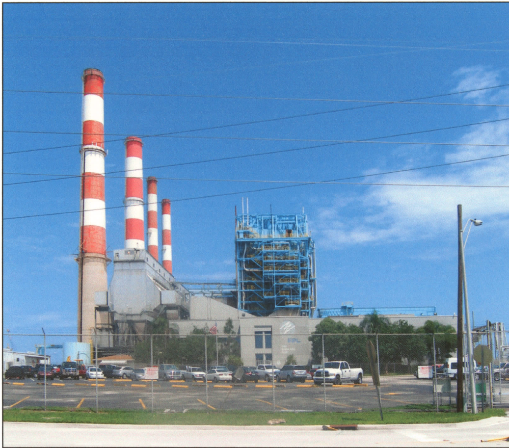
Figure 6. FPL Port Everglades: power plant looking east (entrance).
