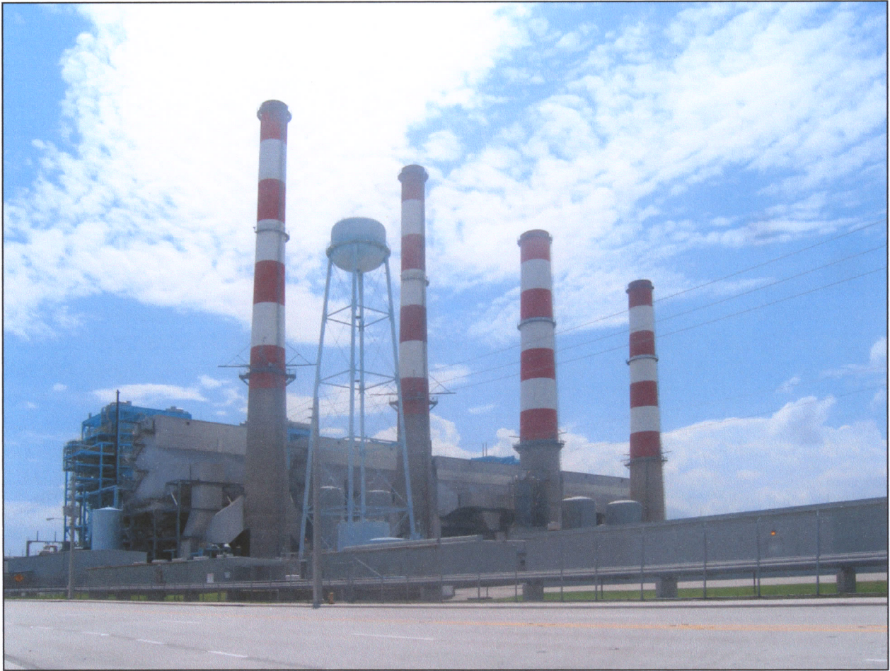
Figure 8. FPL Port Everglades: power plant looking southwest.
