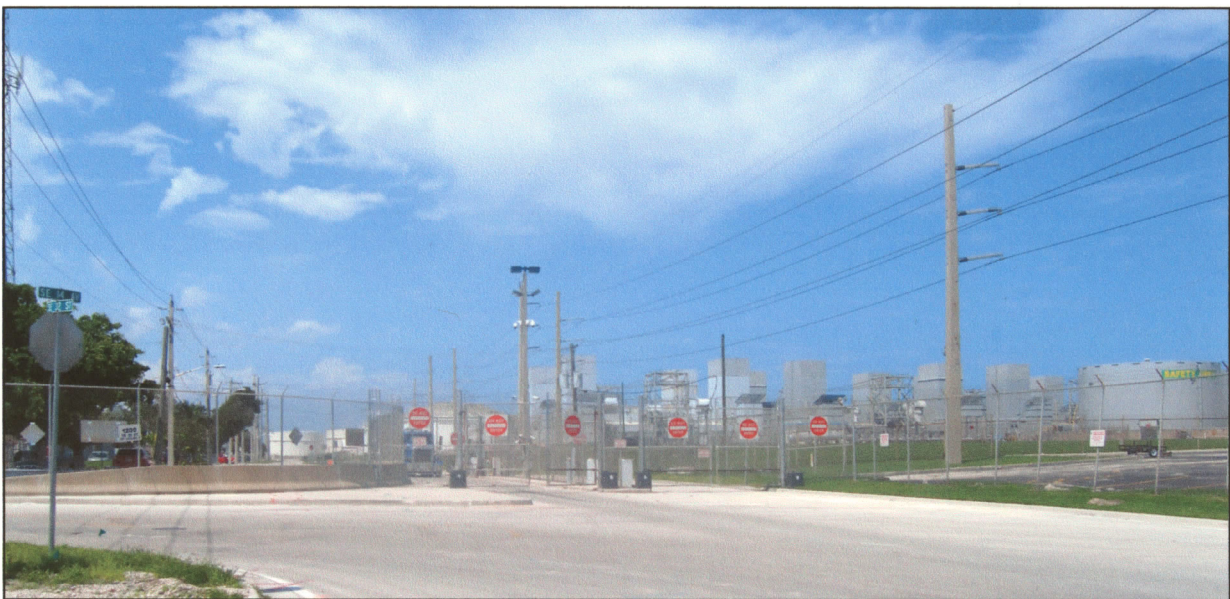
Figure 7. FPL Port Everglades: storage tanks looking northeast.
