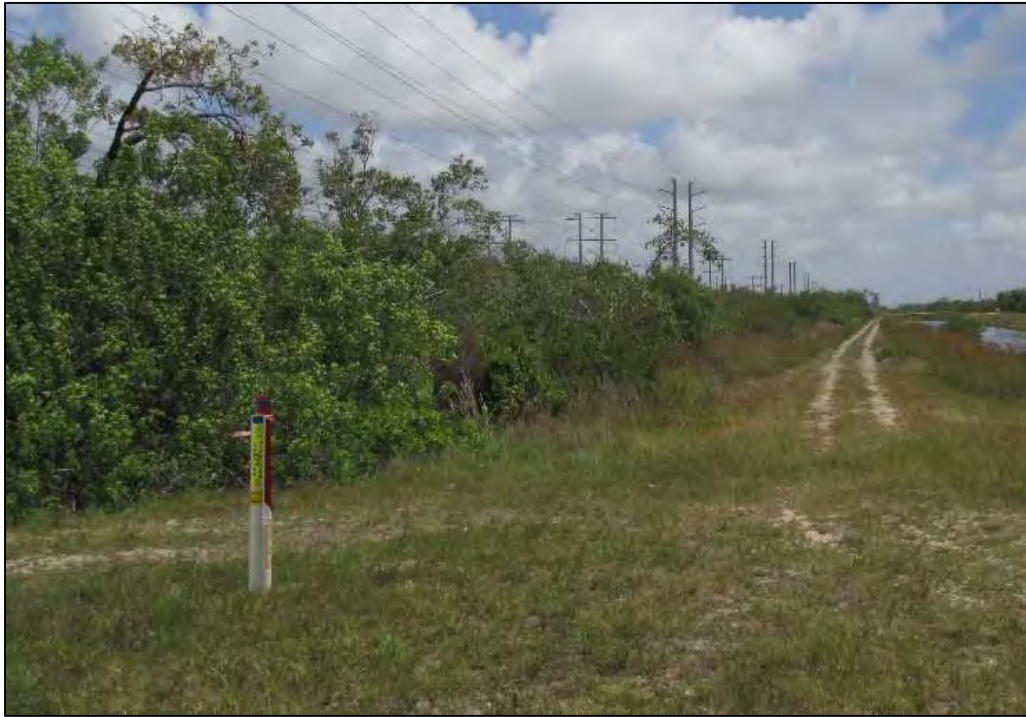
Figure 11: Representative View of Existing Transmission Line Corridor, Filled Patrol Road, Underground Utility Markers, and Adjacent Low Wet Areas within the APE Associated with the CWRC Waterline Corridor, Facing Northwest
