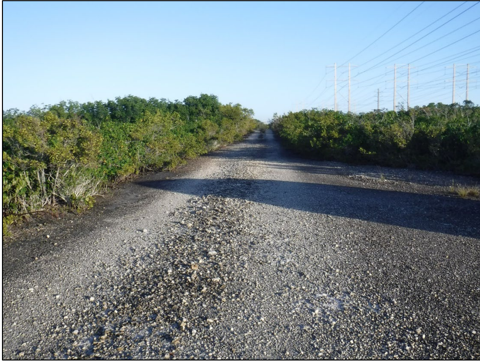
Figure 20: FPL Access Road and Mangrove, Southern Portion of APE, Facing Northwest
