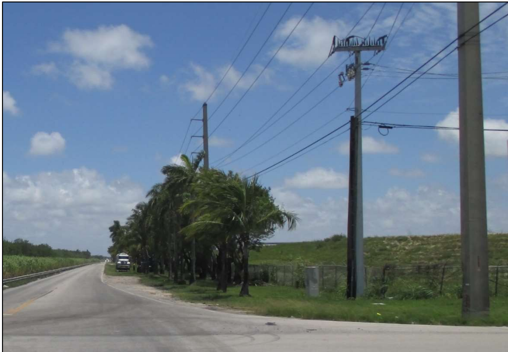
Figure 14: Representative Photograph of Existing Transmission Line Corridor Within a Disturbed Area of the APE Associated with the CWRC Waterline Corridor Adjacent to the Artificially Raised Landfill on the East Side of SW 97 th Avenue, Facing North
