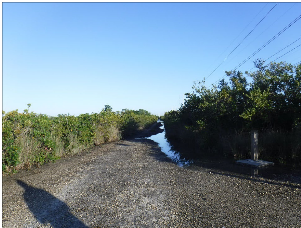
Figure 17: FPL Gravel Access Road and APE, Facing North
