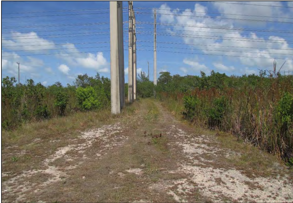
Figure 13: Raised Filled Area of Structure Footer and Adjacent Low Wet Areas of Within the Existing Transmission Line Corridor Containing the Majority of the APE Associated with the CWRC Waterline Corridor, Facing North
