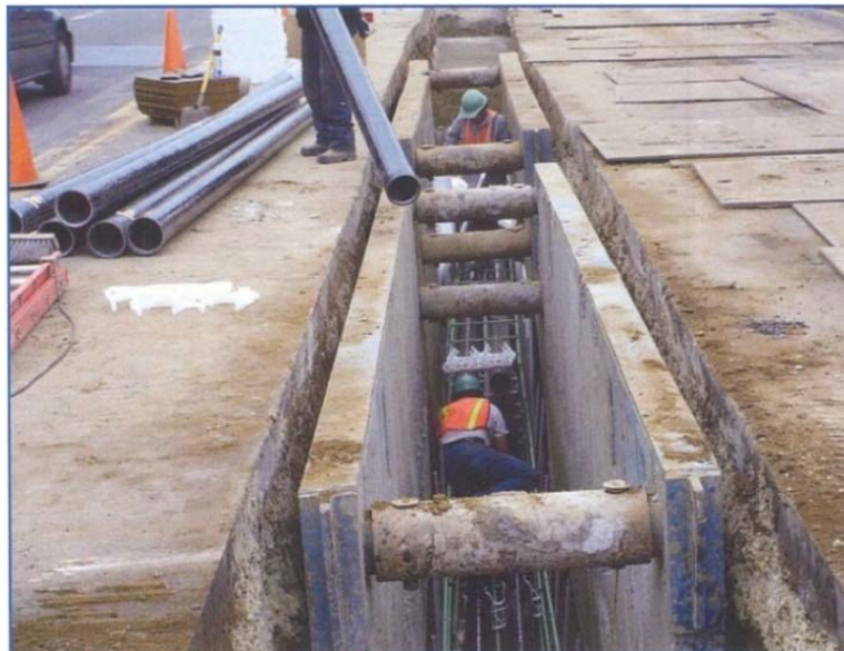
Figure 7 – Construction of Underground Transmission Line (FPL August 11, 2009 presentation to State Representative Lopez-Cantera)
