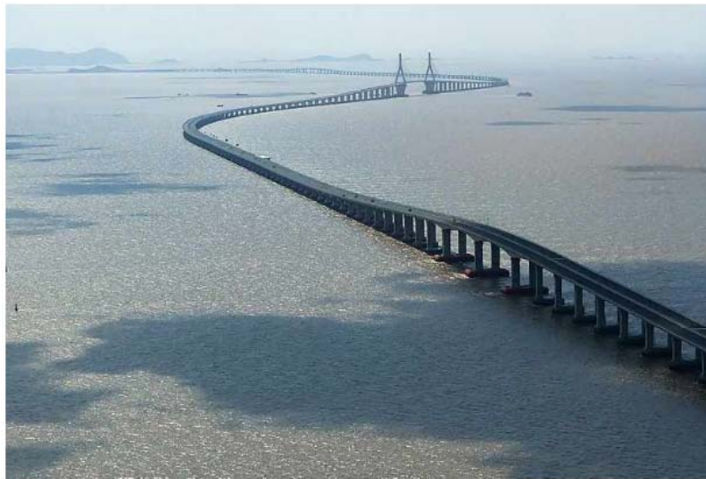
Figure 11 - The Donghai Bridge (photo courtesy of http://steelbuildingshq.com/donghai-bridge/ )
