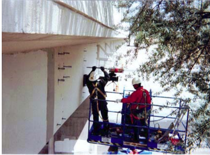
Figure 9 - Typical cable attachment (From Metrorail Attachment Addendum, July 2011)
