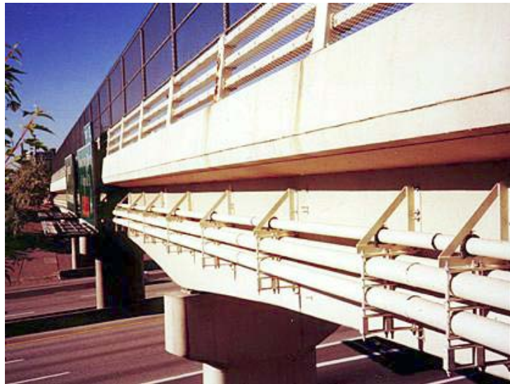
Figure 10 - Typical attachment alongside bridge (From Final Metrorail Attachment Addendum Analysis by FPL, July 2011)
