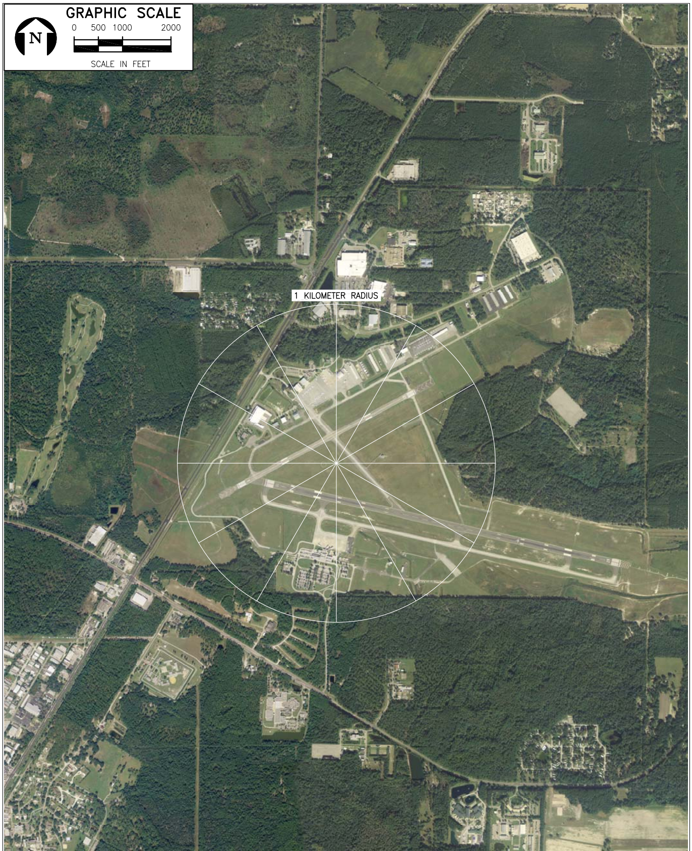
FIGURE 7-6. AERIAL VIEW OF GAINESVILLE REGIONAL AIRPORT
