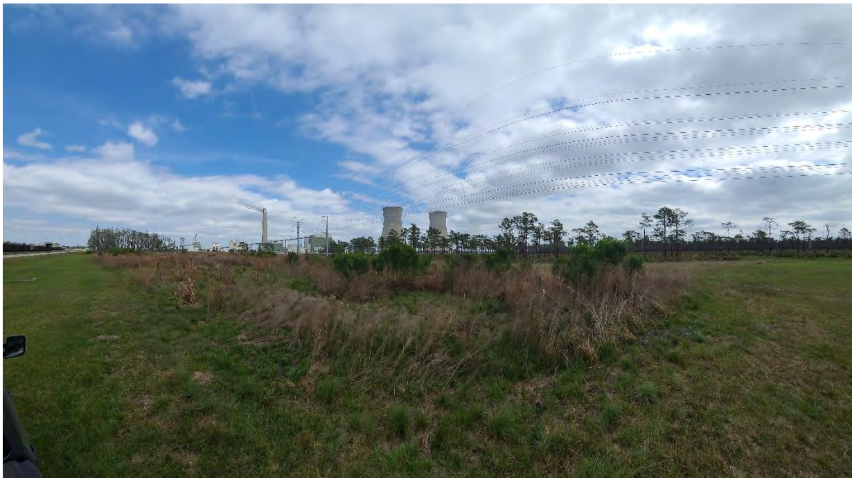
Southeast corner looking northwest - 28^{\circ}28'30.036'' N, 81^{\circ}10'0.876'' W
