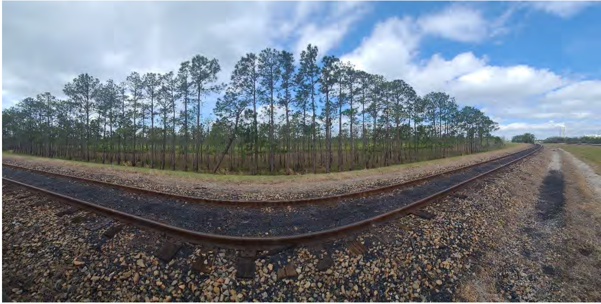
South looking west - 28°28'5.178" N, 81°09'40.5288" W
