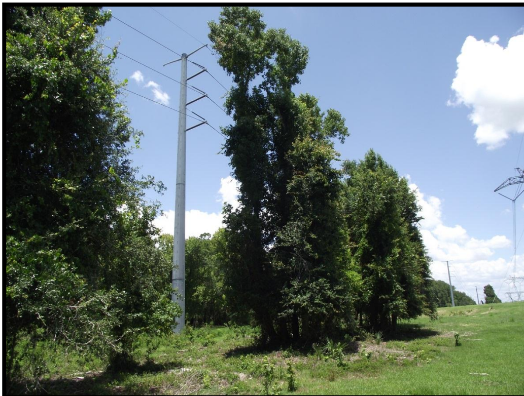
Photo Point 11 - Looking north.
