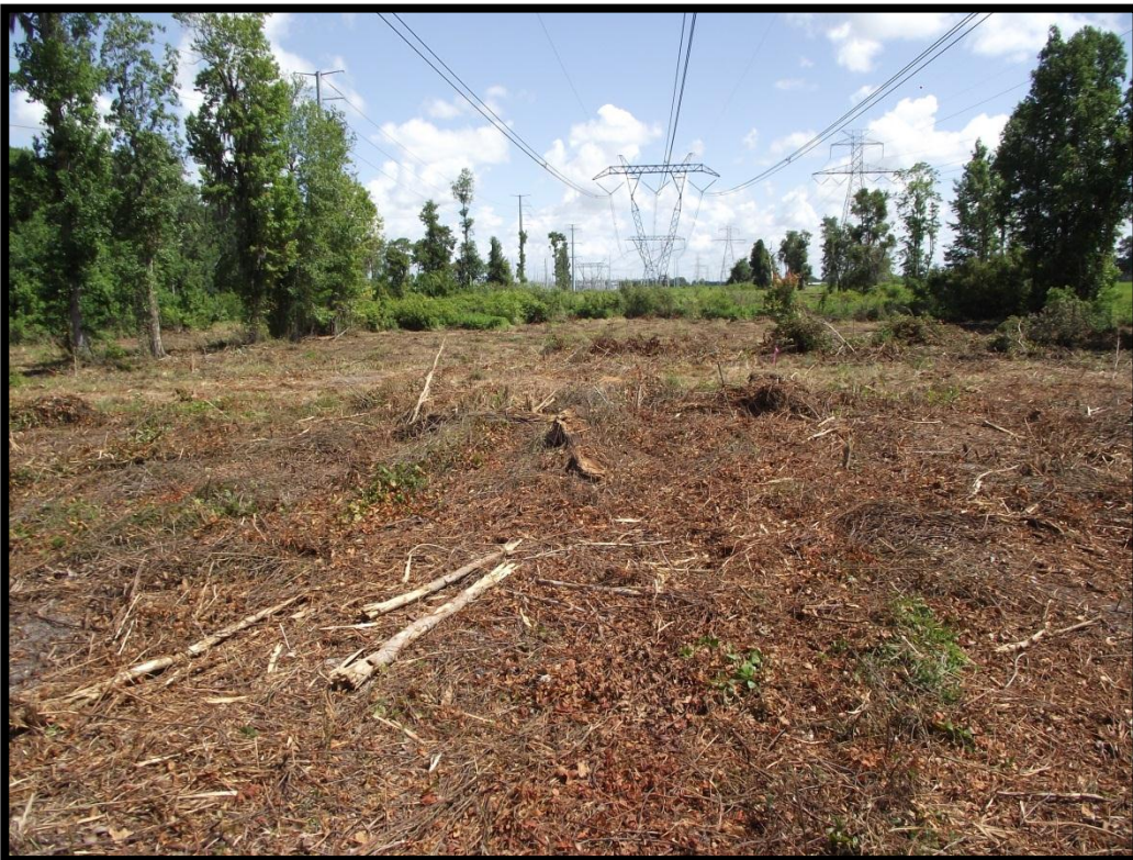
Photo Point 7 – Looking north, recently bush-hogged right-of-way near CFK-4.
