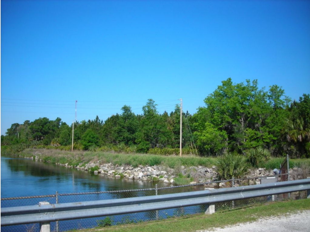
Photograph 1 (above) - View northeast from the Inglis Lock Bypass Channel crossing east of the project providing a view of the location of the proposed access road and bridge.
