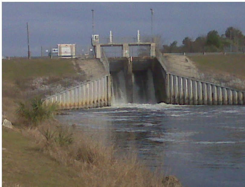
Figure 7. Inglis Bypass Spillway
