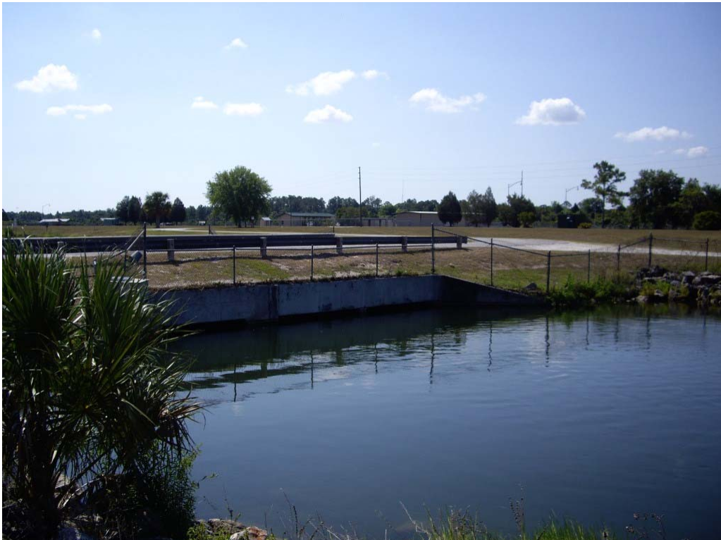
Photograph 2 (below) - View of existing eastern crossing, which has culverts to provide a barrier to navigation.
