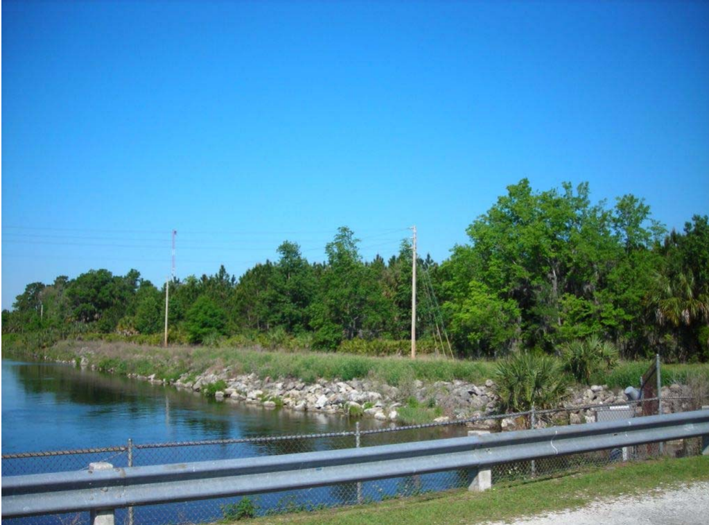
Photograph 1 (above) - View northwest from the Inglis Lock Bypass Channel crossing east of the project providing a view of the location of the proposed access road and bridge.
