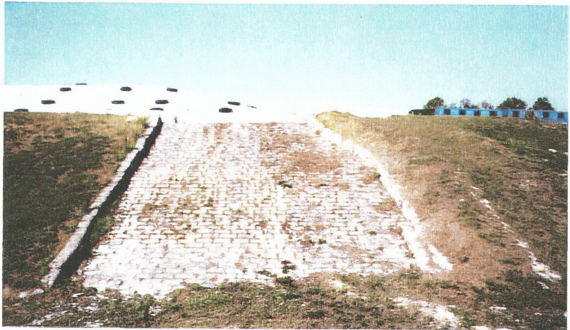
Cemented Bag Spillway - Figure 6
