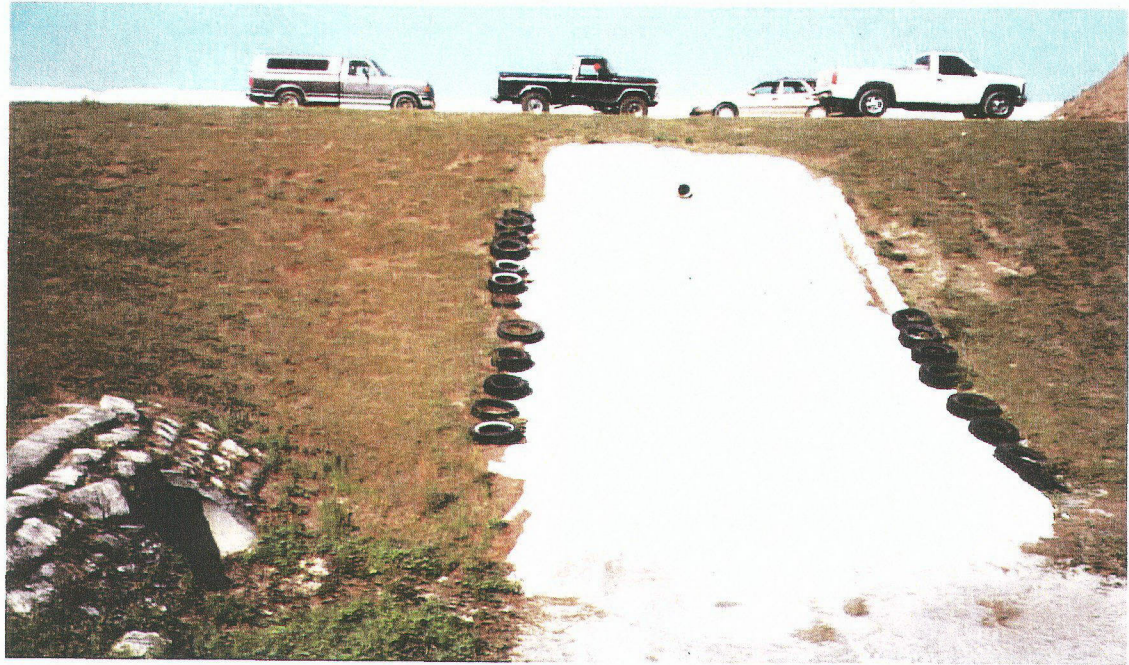
Rain Tarp Spillway - Figure 5
