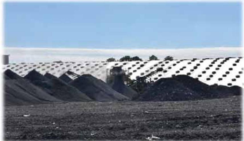
Figure 6-2 Segregated Aggregate Piles
