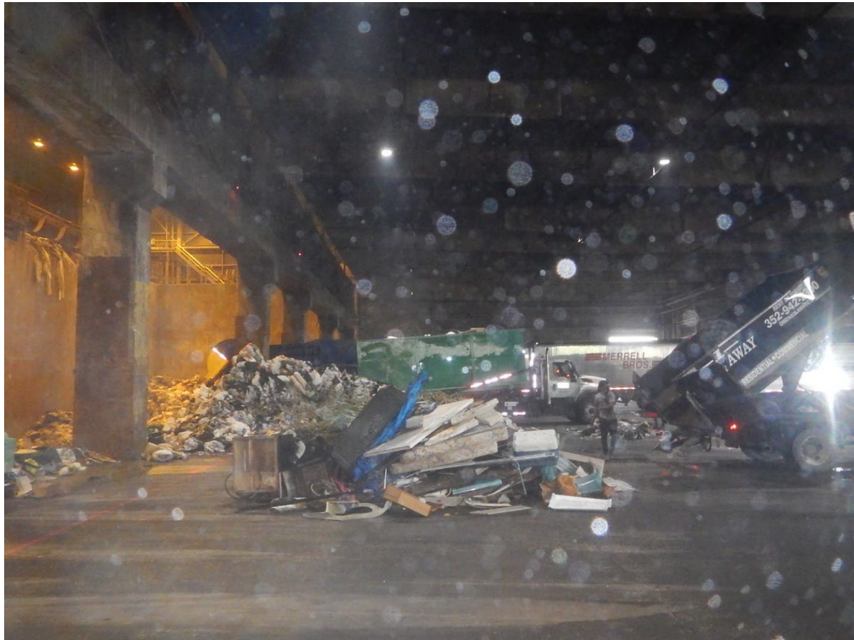
Figure 3-2. MSW Deposited on the Tipping Floor, with the Refuse Storage Pit to the Left
