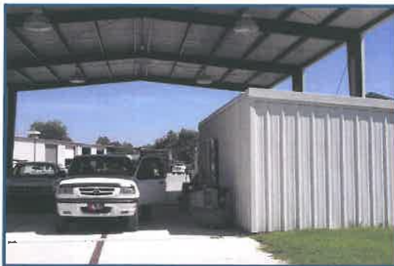
Figure 8. Example of heavy equipment washing facility equipped with a 100% closed-loop recycle system.
