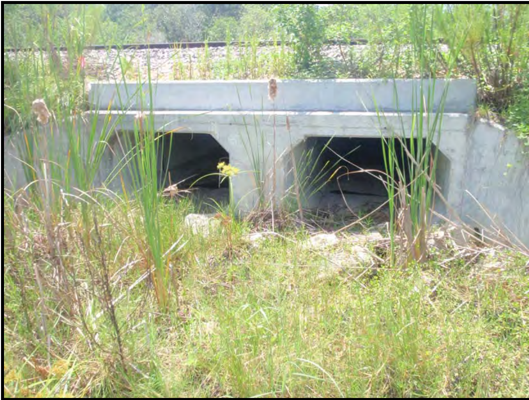
Photograph No. 17. View of culverted railroad crossing which drains Wetland W1 looking west from edge of Wetland W1.
