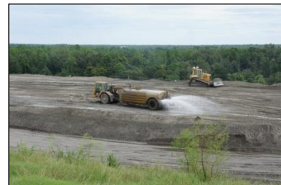
Water Wagon and Dozer Active Disposal Area
