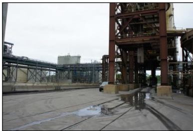
Unit 4 Bottom Ash Silos
