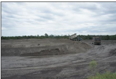
Fly Ash Placement
