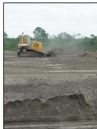
Spreading Fly Ash
